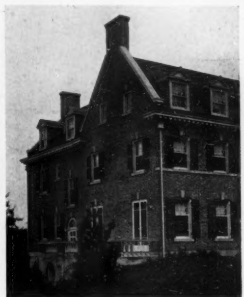
It is common practice in Colonial work to carry up the chimney flush with the wall
