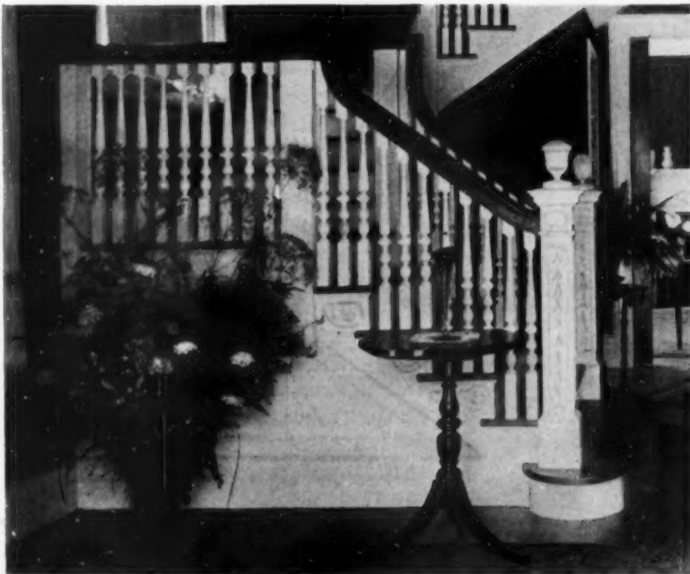
It usually results in a better appearance and requires less space to change the direction once or twice rather than having a straight run
