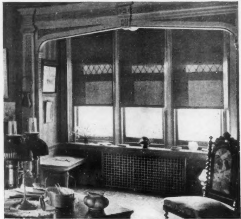
It is possible often to conceal the radiators of Steam or Hot Water systems under a seat
