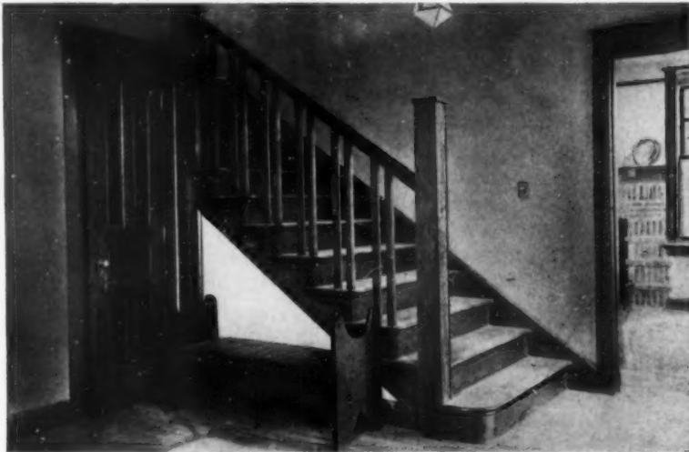
A very simple and inexpensive form of stairway that would be well suited to a house of the craftsman type. W. D. Brincklé, architect
