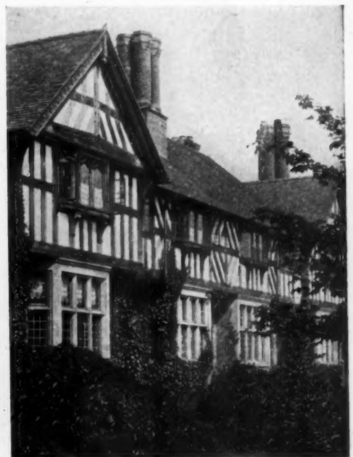
On half-timber work the chimneys are usually of an intricate pattern in brick or terra cotta
