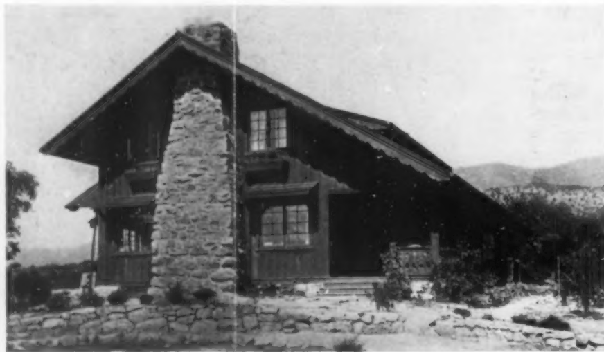
A massive stone chimney, with a fireplace measuring ten feet across the chimney breast, distinguishes one end of the building
