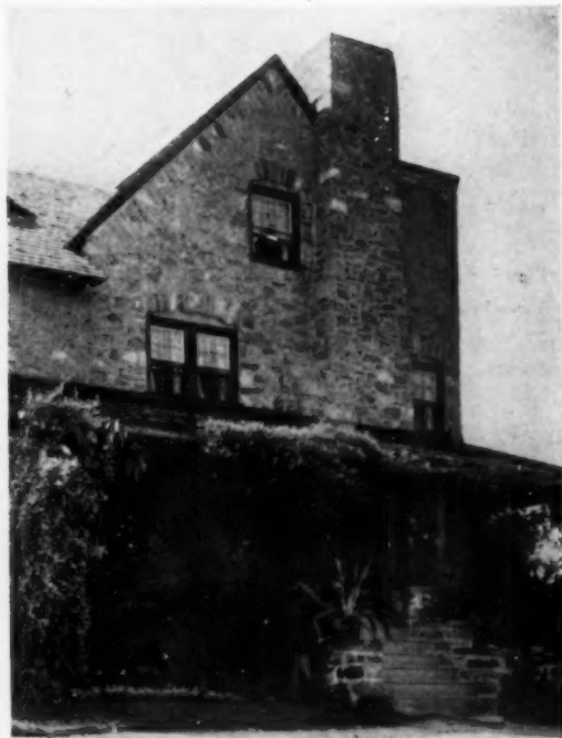
A stone chimney that composes particularly well with the gable end of which it is a part
