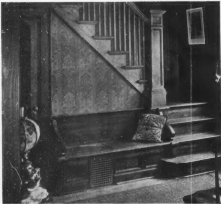
An example of careful planning in the location of a register in a Hot Air system
