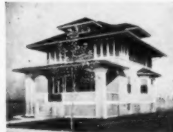
A No. 3-22 IDEAL Boiler and 600 ft. of 38-in. AMERICAN Radiators, costing the owner $255, were used to Hot-Water heat this cottage.
