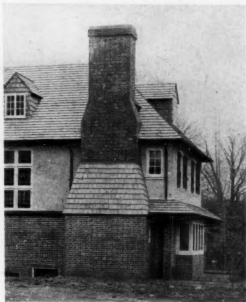
A chimney of common bricks, laid Flemish bond, that seems particularly appropriate
