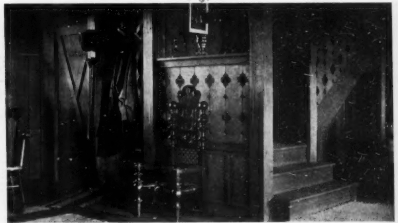
The effective woodwork that takes the place of the balustrade is made of pine boards with a sawed-out pattern
