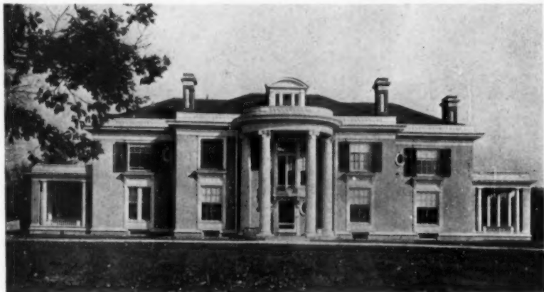
Here the chimneys are of brick with inset plaster panels and cornices to match the gray plaster of the walls
