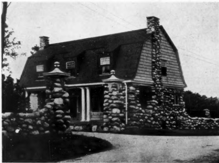
In a gambrel roof the most appropriate dormers have for their roofs a continuation of the upper slope
