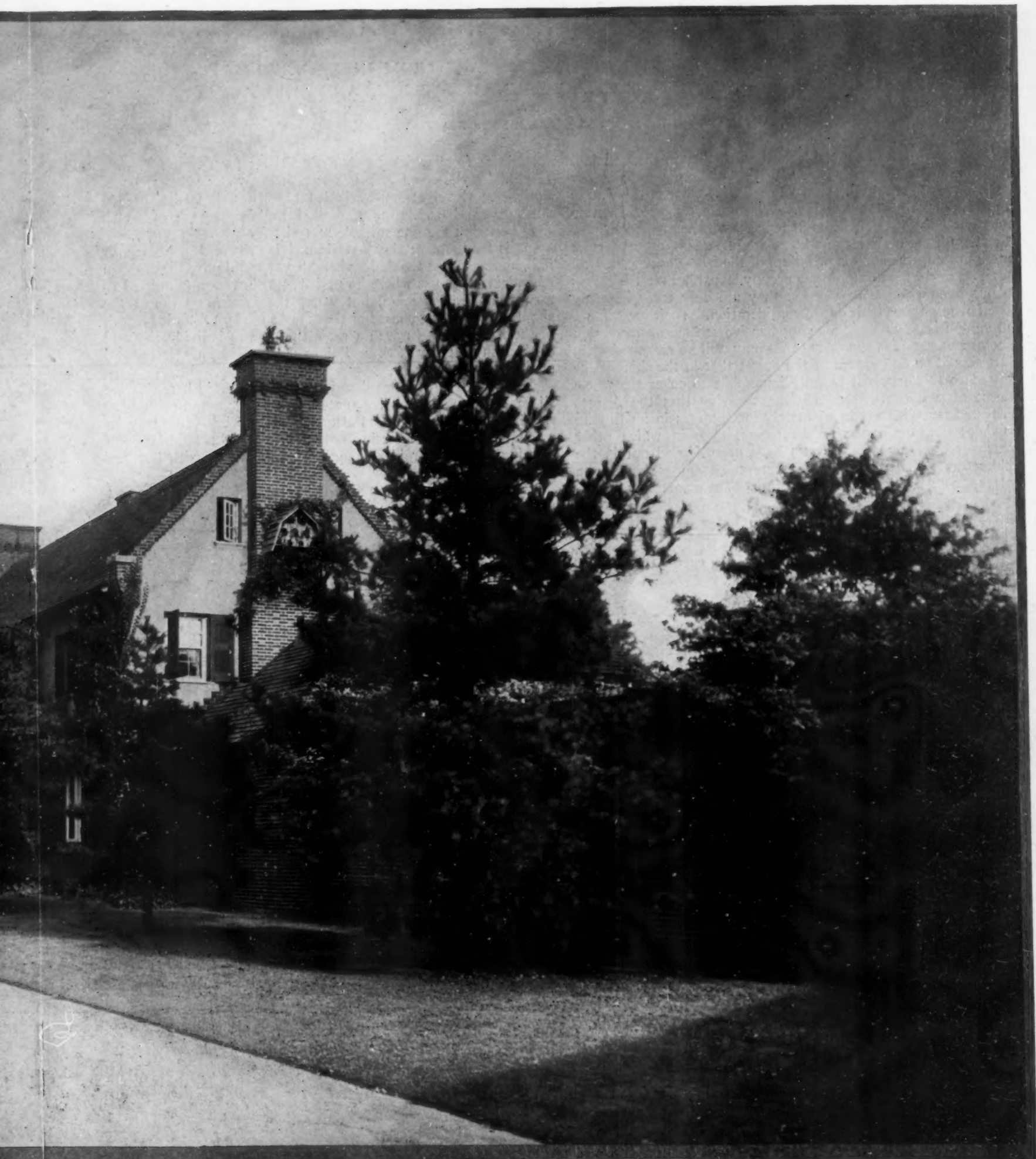
PHOTOGRAPH BY MR. THOMAS W. SEARS, LANDSCAPE ARCHITECT WHAT CAN BE DONE IN AMERICA IN A FEW YEARS—THE BORIE HOUSE, RYDAL, PA., MR. WILSON EYRE, ARCHITECT
