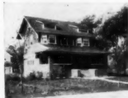
A No. 3015 IDEAL Boiler and 775 sq. ft. of 38-in. AMERICAN Radiators, costing the owner $125, were used to Steam heat this cottage.
