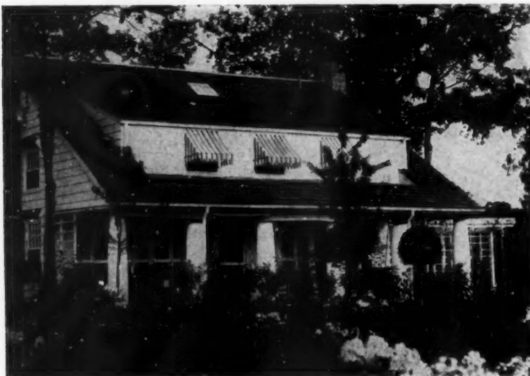
A continuous dormer gives more space in the upper story. Chauncy Olcott's home, Saratoga. Keen & Mead architects
