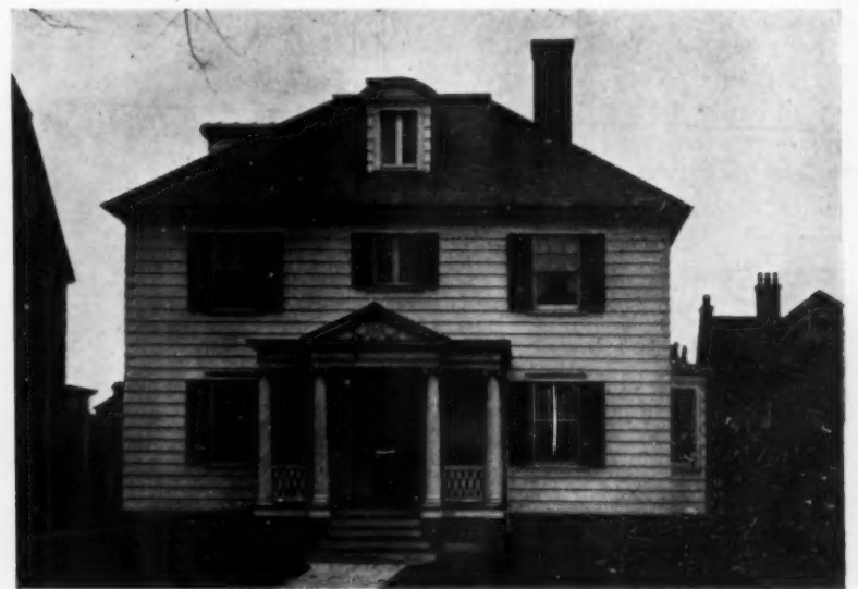
The rounded-top dormer, as on this Rochester house, is not very common in modern work. Claude Bragdon, architect
