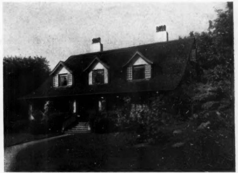
These broad, high-gabled dormers would be out of place on any roof other than one with such a broad low sweep
