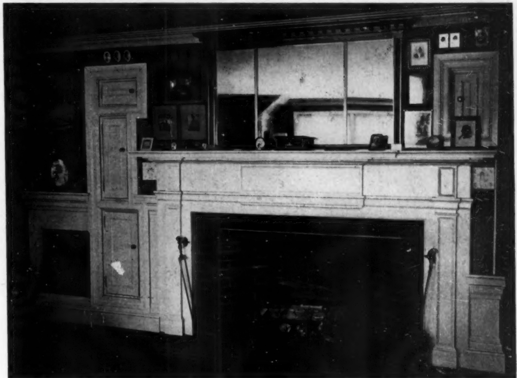
The type of mantel that distinguishes the genuine Colonial architecture. A mirror of this kind is not easily improved upon for the over-mantel decoration
