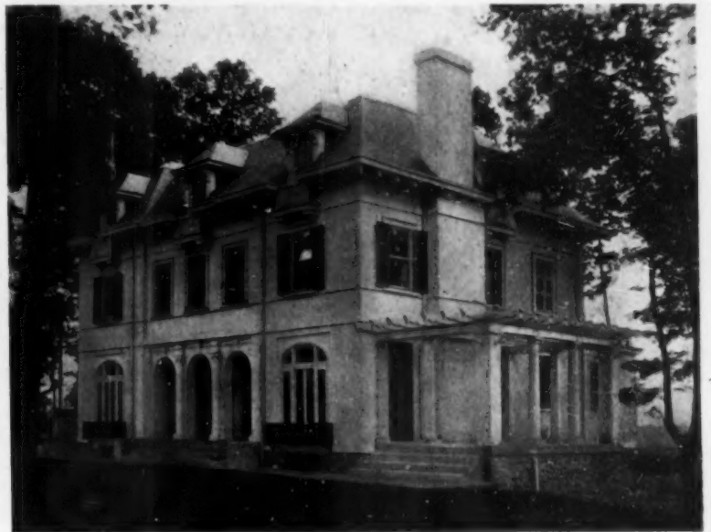
These dormers are somewhat unusual in that they break through the eaves. Ellicott & Emmart, architects
