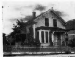
A No. 3-22 IDEAL Boiler and 400 sq. ft. of 38-in. AMERICAN Radiators, costing the owner $215, were used to Hot-Water heat this cottage.
