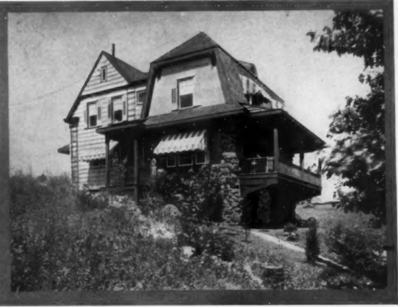
The kitchen and service porch are at the left, conveniently near the street front
