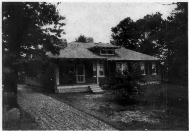
For the walls and roof cypress shingles have been used, not stained but left to weather
