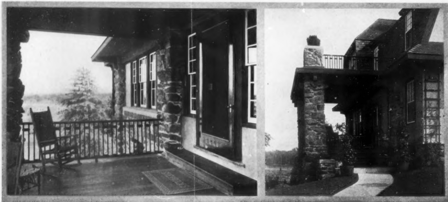
The entrance porch, 13x20 ft., is on the north side of the house, convenient to the corner of the two streets, and marked by massive stone piers.
