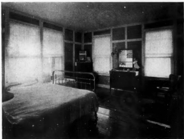
Over the inside sheathing strips of white-painted cypress divide the wall space into panels
