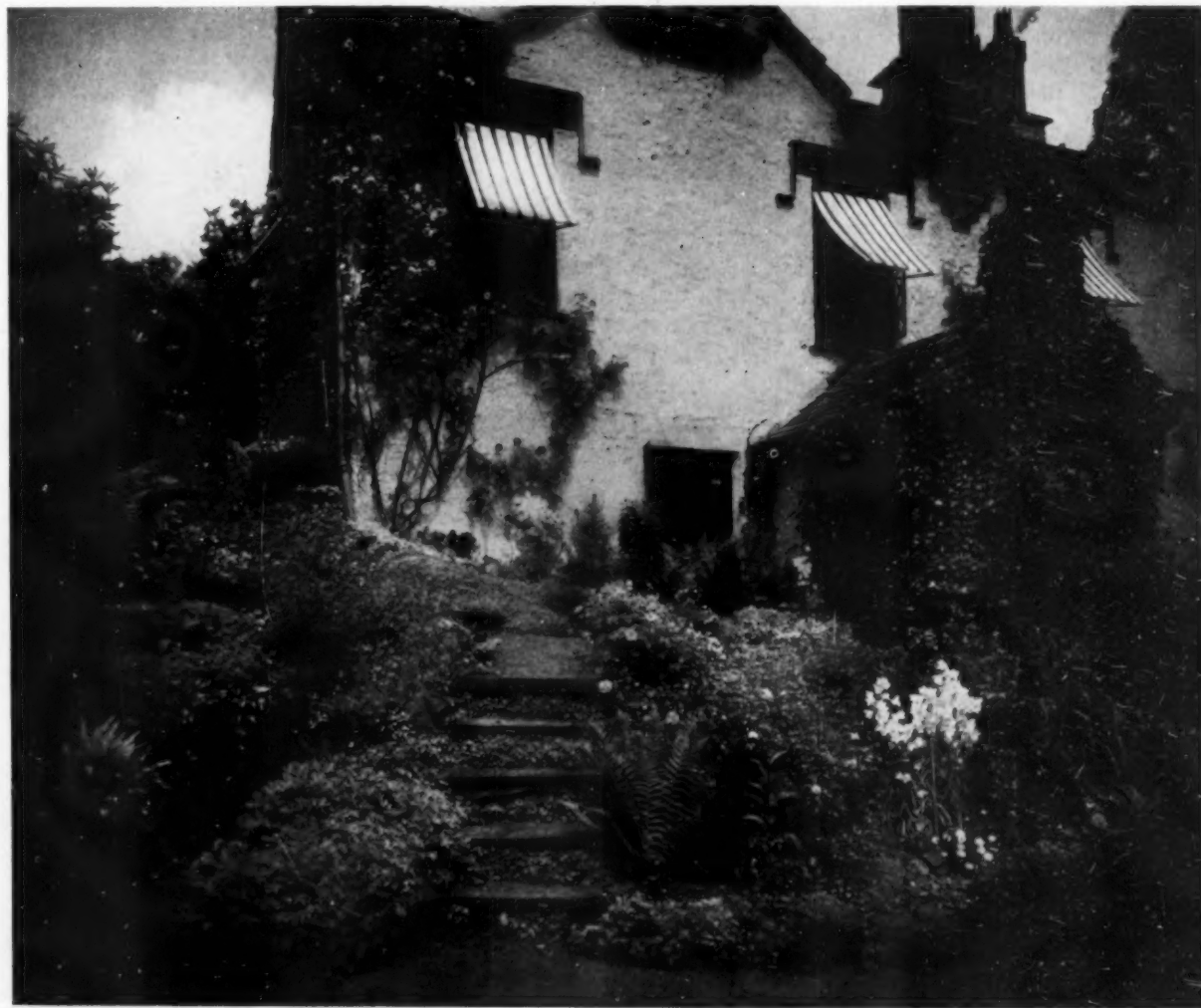
Here is a convincing argument against "grading" a hilly site
