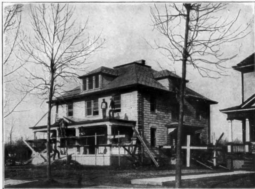
Illustrating a Concrete Block House of Dr. H. C. Howard, Champaign, Illinois, Prof. F. M. White, Architect, roofed with Asbestos "Century" Shingles, laid French Method.
