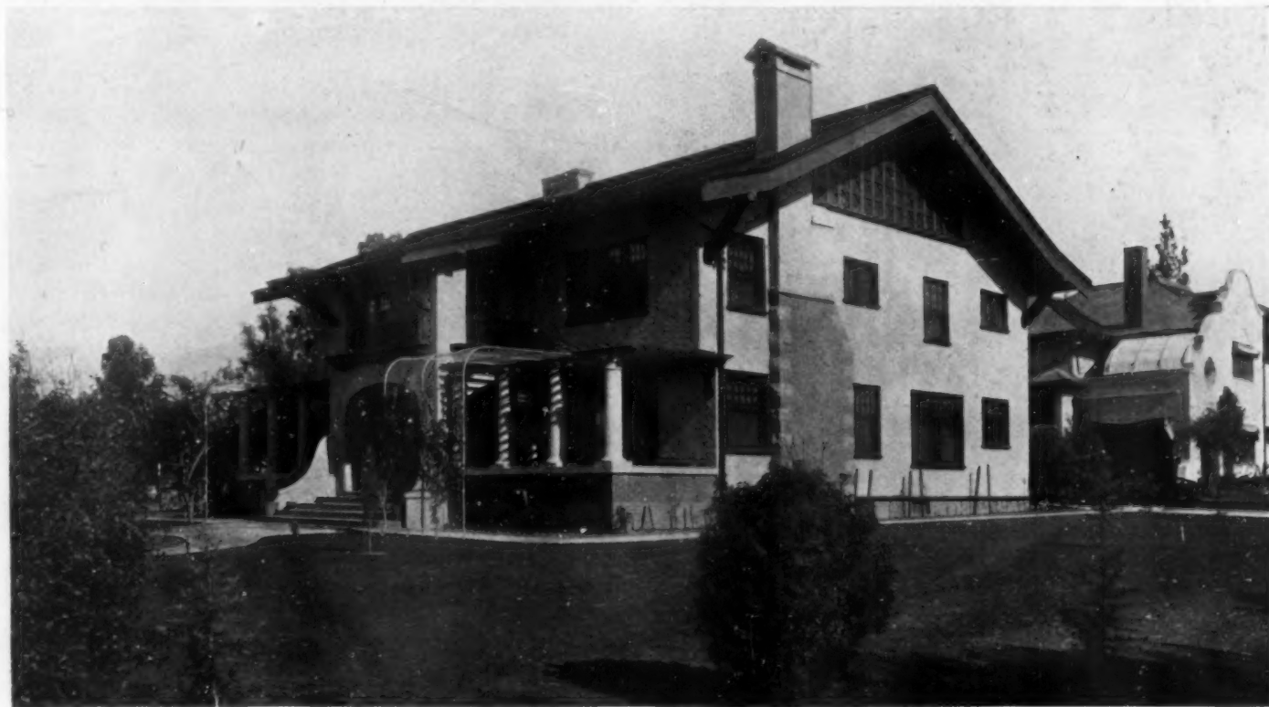
THE HOUSE OF W. C. BAKER, ESQ., PASADENA, CALIFORNIA. SPATTER-DASH STUCCO ON METAL LATH
