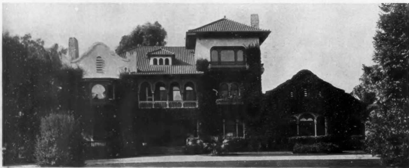
RESIDENCE OF L. V. HARKNESS, ESQ., PASADENA, CALIFORNIA. STUCCO ON METAL LATH
