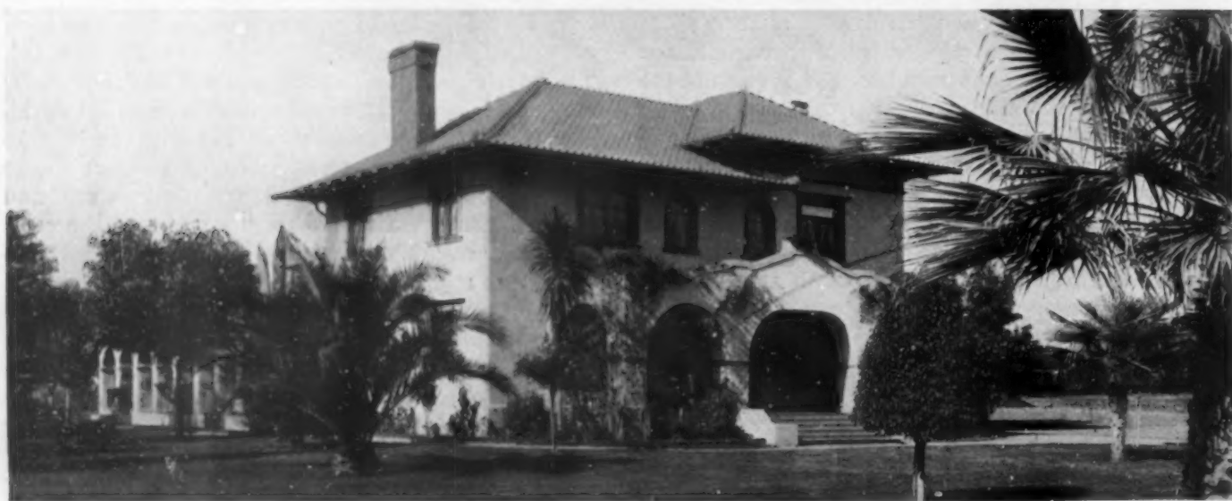
HOME OF FRANK W. EMERY, ESQ., PASADENA, CALIFORNIA. STUCCO ON METAL LATH
