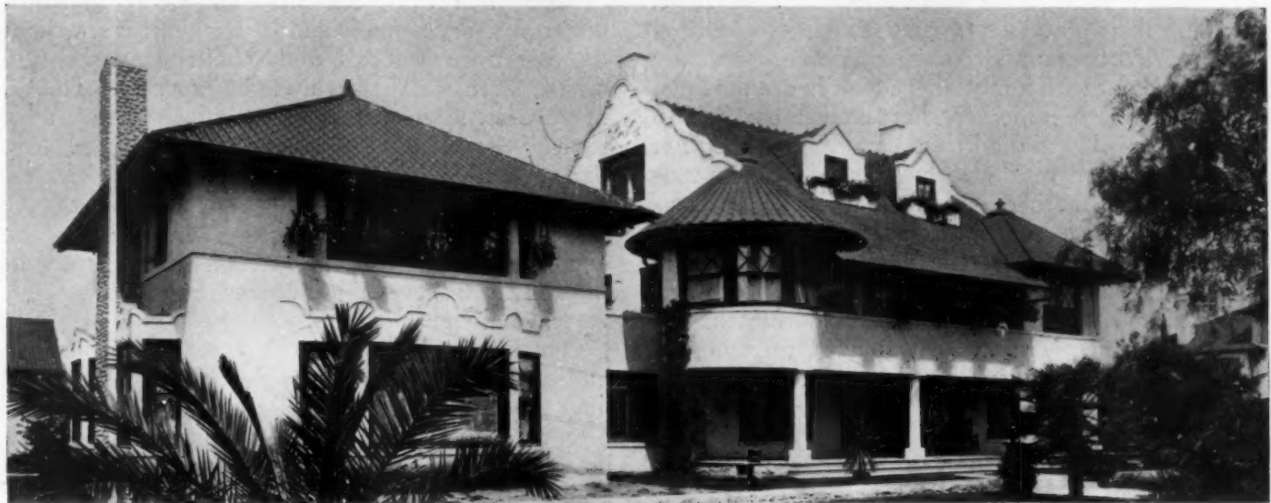
HOUSE OF H. T. KENDALL, ESQ., PASADENA, CALIFORNIA. STUCCO ON METAL LATH
