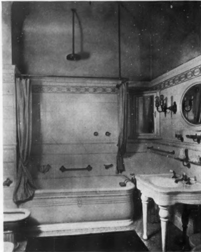
A modern bath-room with square, six inch wall tile to a height of seven and a half feet. Walls above and ceiling painted in flat finish oil colors
