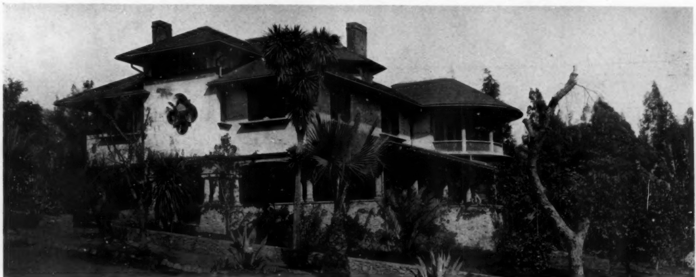
HOUSE OF D. M. SMYTH, ESQ., PASADENA, CALIFORNIA. STUCCO ON METAL LATH
