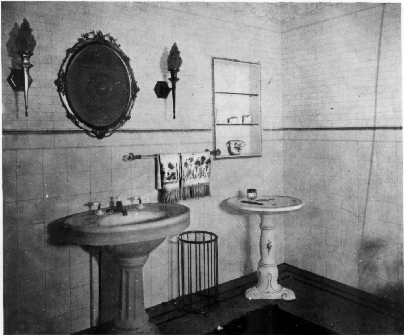
Bath-room with ceramic mosaic floor and walls tiled to ceiling. Tiled recess with glass shelves for toilet accessories
