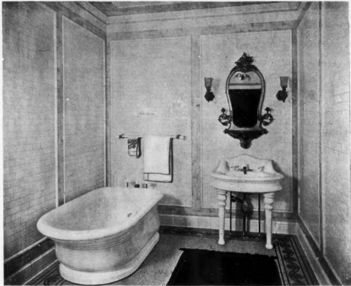
Illustrating cove base tile, with ceramic mosaic floor and the use of panels of tile on walls and ceiling
