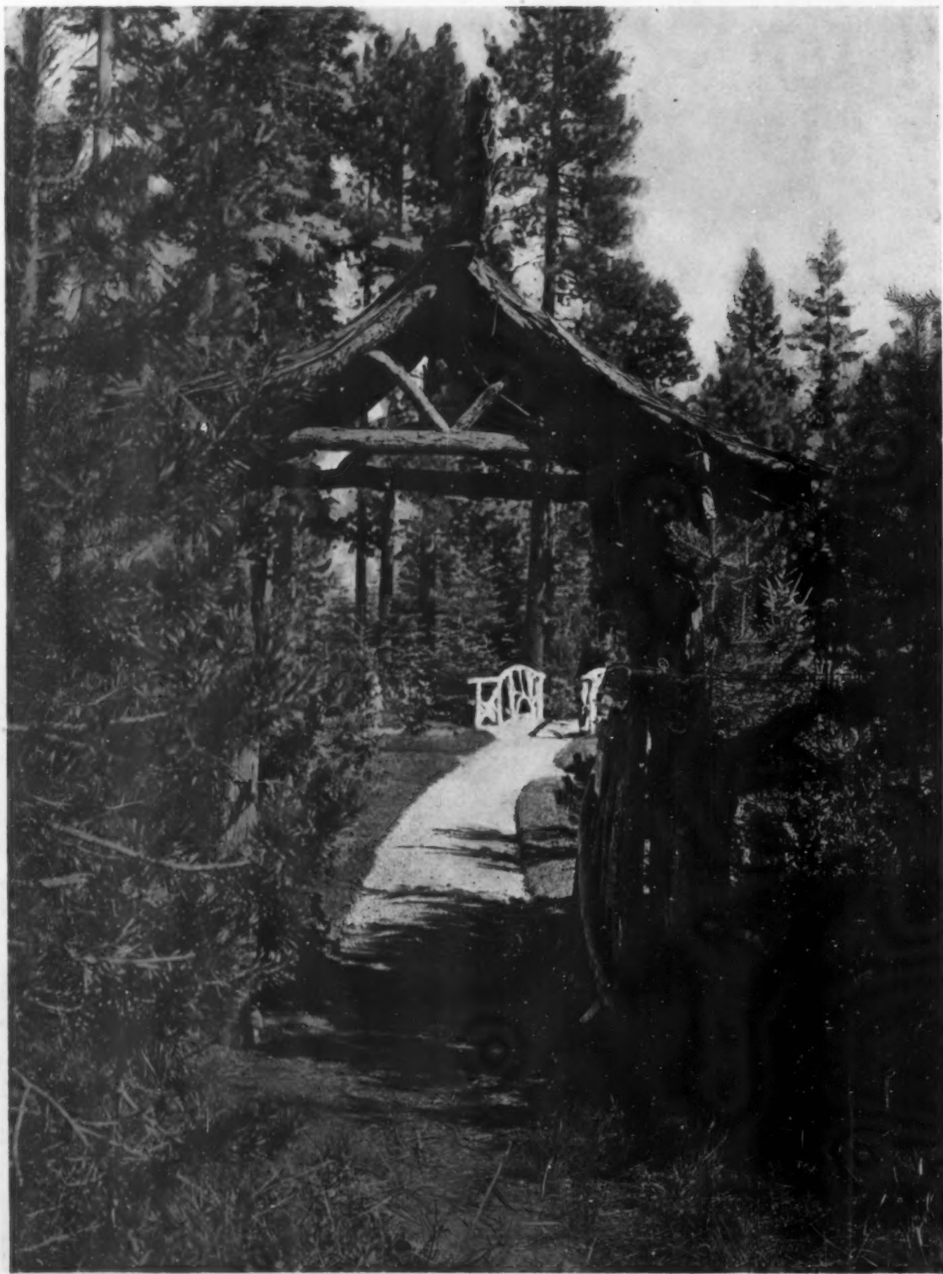
THE ENTRANCE TO THE PRIVATE GROUNDS OF "AROHEAD"
