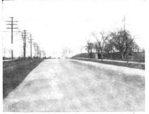
Newton Boulevard, near Boston, made dustless with "Tarvia." Results after the first winter showing smooth hard surface free from loose stone or dust.
