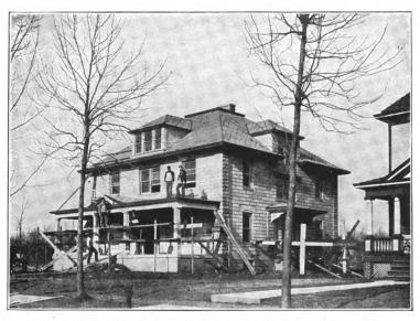
Illustrating a Concrete Block House of Dr. H. C. Howard, Champaign, Illinois, Prof. F. M. White, Architect, roofed with Asbestos "Century" Shingles, laid French Method.
