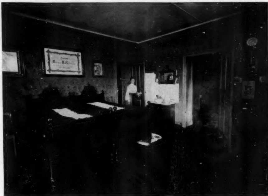
BEDROOM OF A FOREMAN'S DWELLING—COLONY WILDAU
