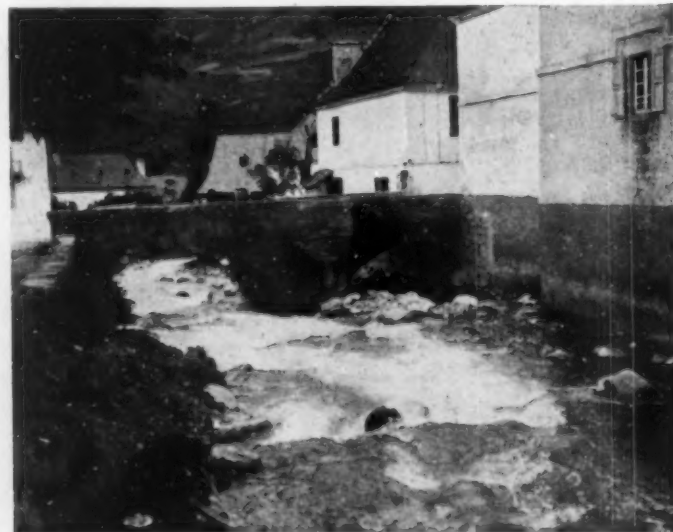
Bridge at Viella
