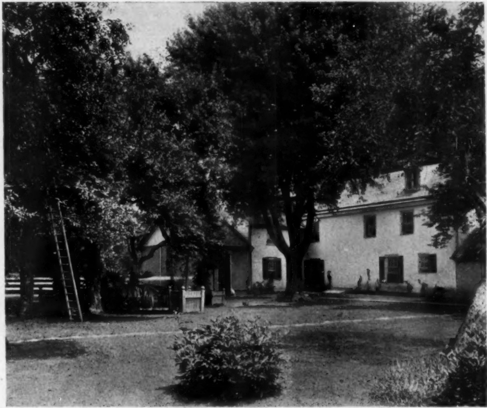
THE KITCHEN ENTRANCE
