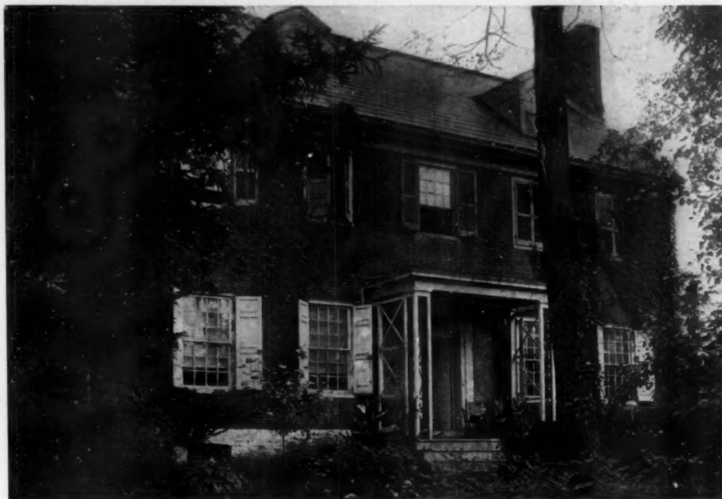
THE ENTRANCE TO THE HOUSE
