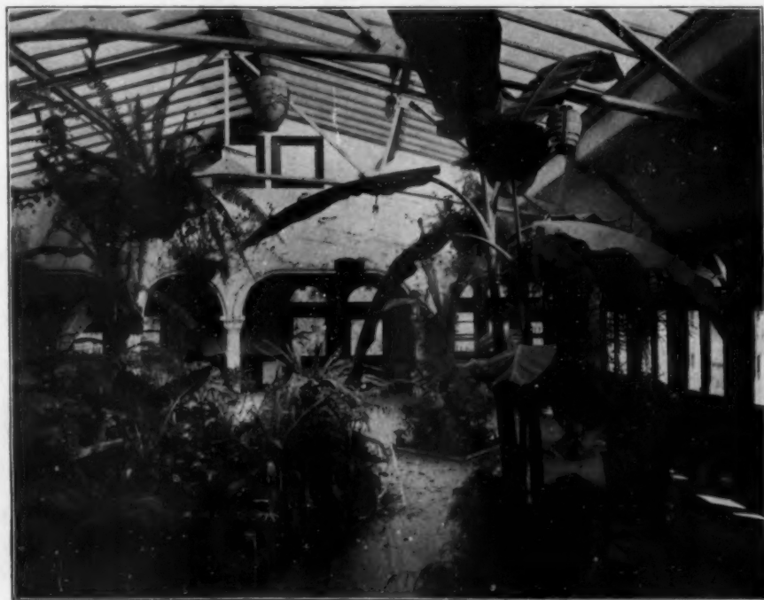
A COVERED PATIO
