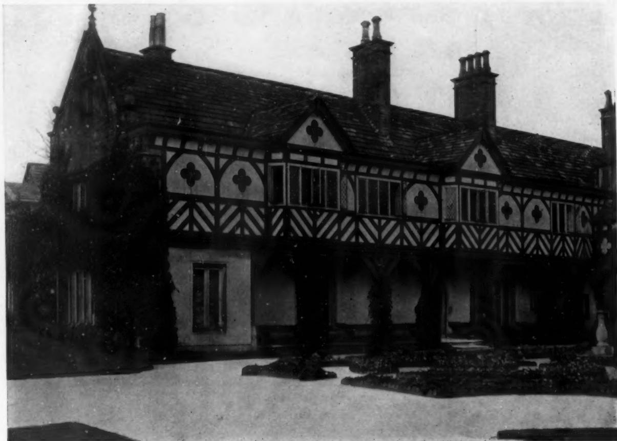
THE RECONSTRUCTED VERANDA
