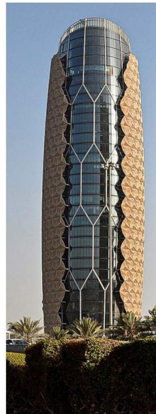
Al Bahr Towers designed by the London offices of Aedas and Arup
