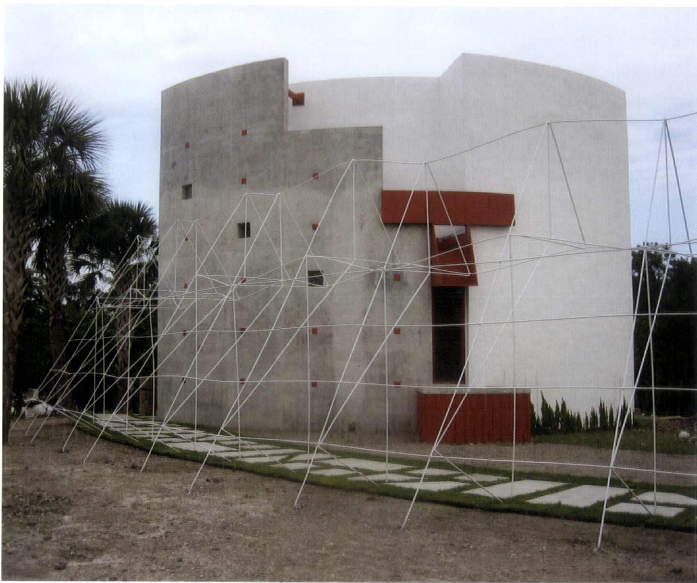
Above: South elevation of the guesthouse. Behind the exposed concrete wall is the stair to the second floor. The roof of this stair works as a fountain that re-circulates water to a tank on the ground. The red dots are ceramic inserts for decoration.
