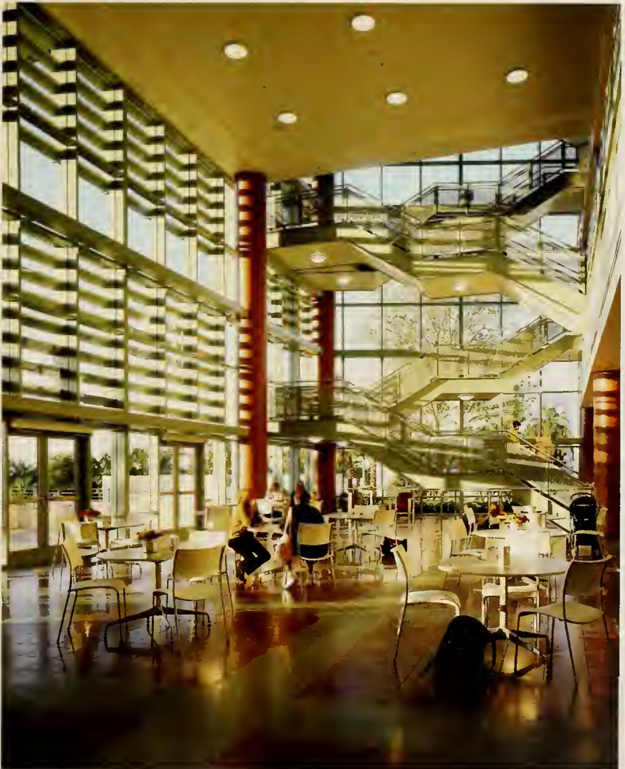
Light enters the building through solar deflecting blades thus reducing the need for artificial light. Photos: top, materials area, and below, the grand staircase. All photos by George Cott, Chroma.
