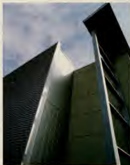
Compressor blade replica detail with stair tower clad in corrugated metal.
