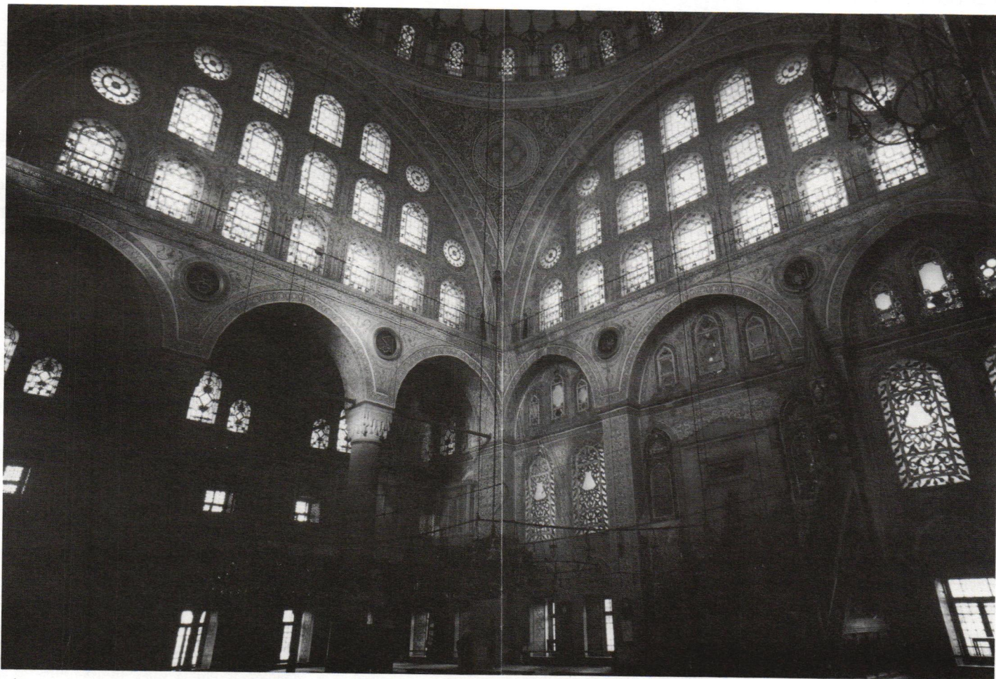
In the mosque of Süleyman's daughter, Princess Mihrimah, Sinan eliminate corner piers, relegating them to the outside of the mosque. The dome rests on four pendentives, which seem to melt away in the light flooding from walls that no longer support any weight. The dome appears suspended, like the canopy of Heaven. (From Sinan .)
