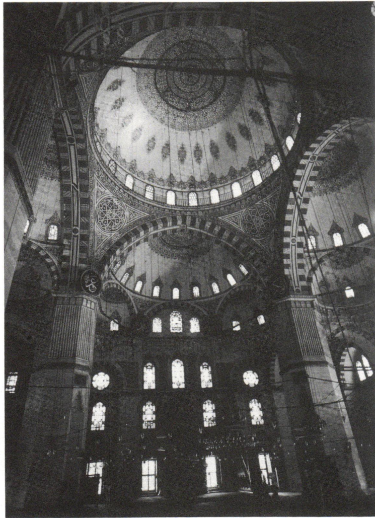
In the Şehzade [sic] Mehmet Camii, Sinan took the plan of Hagia Sophia to its logical conclusion. Instead of building two semidomes to support the central dome, he erected four, creating a perfect symmetry. (From Sinan .)
