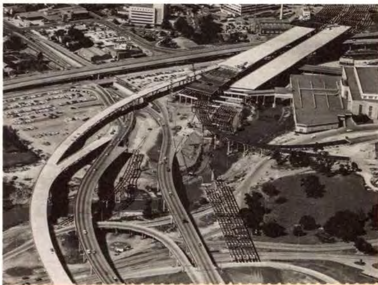
030 Houston: Construction of IH 45 elevated section
