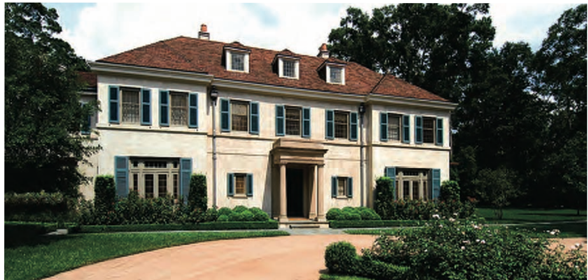
House 1 Entrance court—the porch is cast concrete, the walls are acid-washed stucco.
