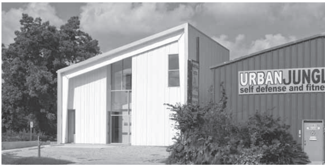
Front façade showing pre-engineered structure and vertical siding.
