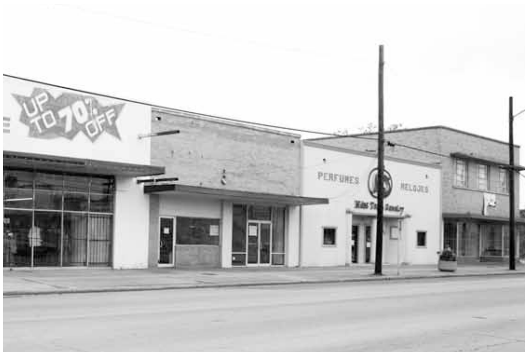
Box 13 ArtSpace, corner lot, Harrisburg and Cesar Chavez boulevards.
