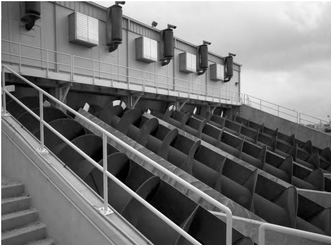
Enhanced versions of the Archimedean screw can lift 125,000 gallons of water per minute over an 11-foot barrier.
