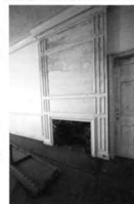
Opposite page, top: To get to the original plantation house (right), outbuildings had to be stripped away (left). Opposite page, bottom: Two generations of the Dew family in front of their homestead, circa early 20th century. Top: Dew Plantation House, 1901 Bottom: Interior fire place, 2006.
