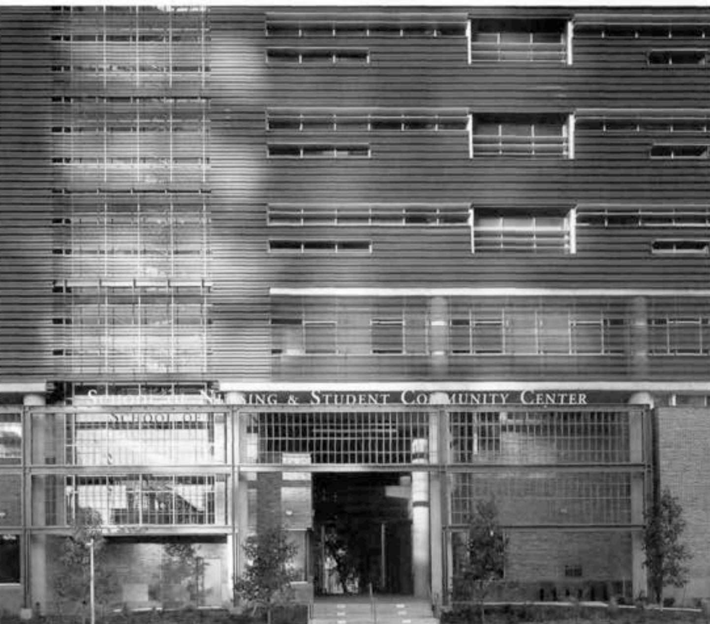
Perforated metal siding adds depth and shading to the School of Nursing Building's west side.
