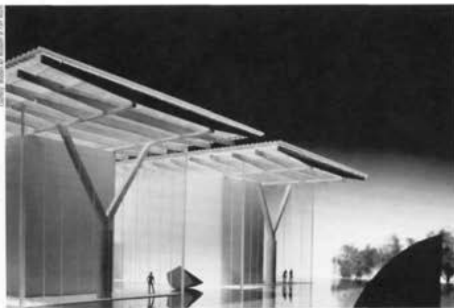
Ando's competition rendering revealed a light-filtering roof, intended to be realized in glass and steel.
