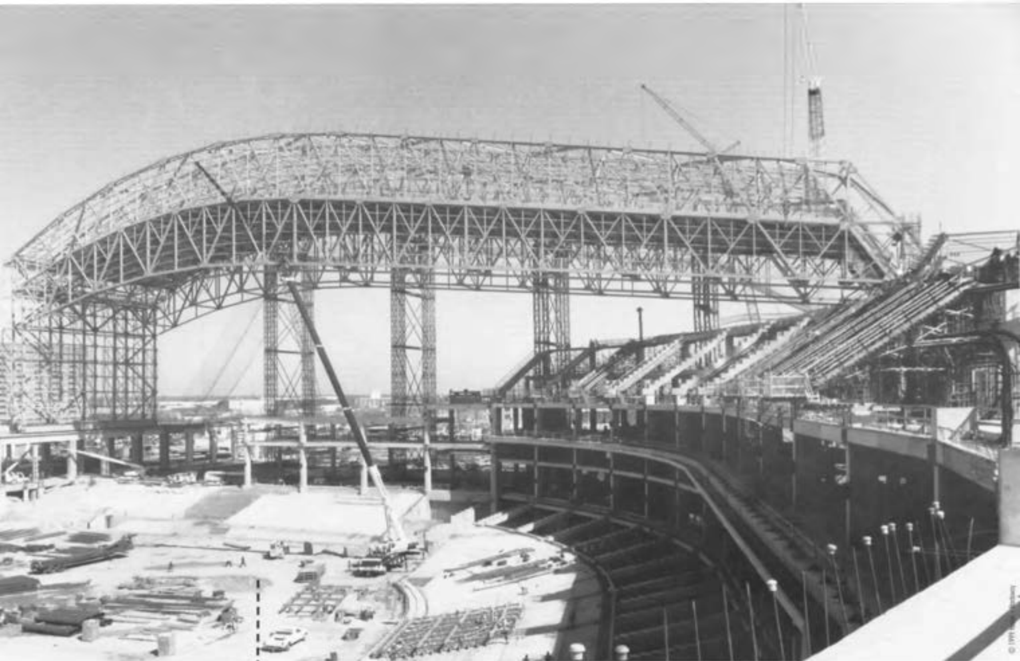
When completed, the retractable roof of the Ballpark at Union Station will, at its highest point, rise 242 feet above the playing field — 38 feet higher than the highest point in the Astrodome.
