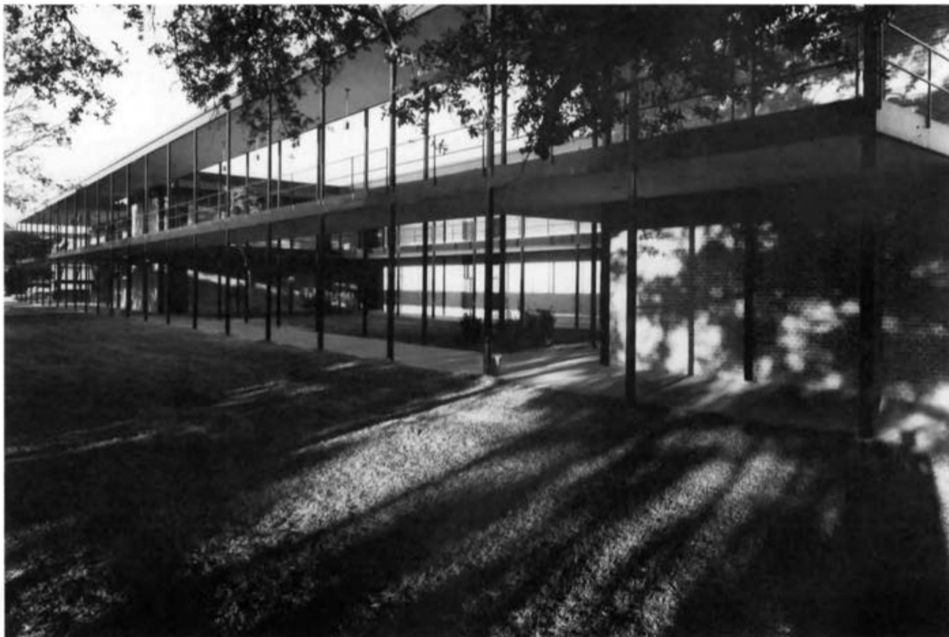
University of St. Thomas academic court showing Jones and Strake halls connected by the two-story arcade, Philip Johnson, architect (1958-59).
