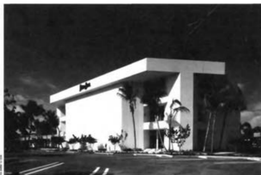
Neiman Marcus, Bal Harbour, Florida, Herbert H. Johnson, architect (1971).
