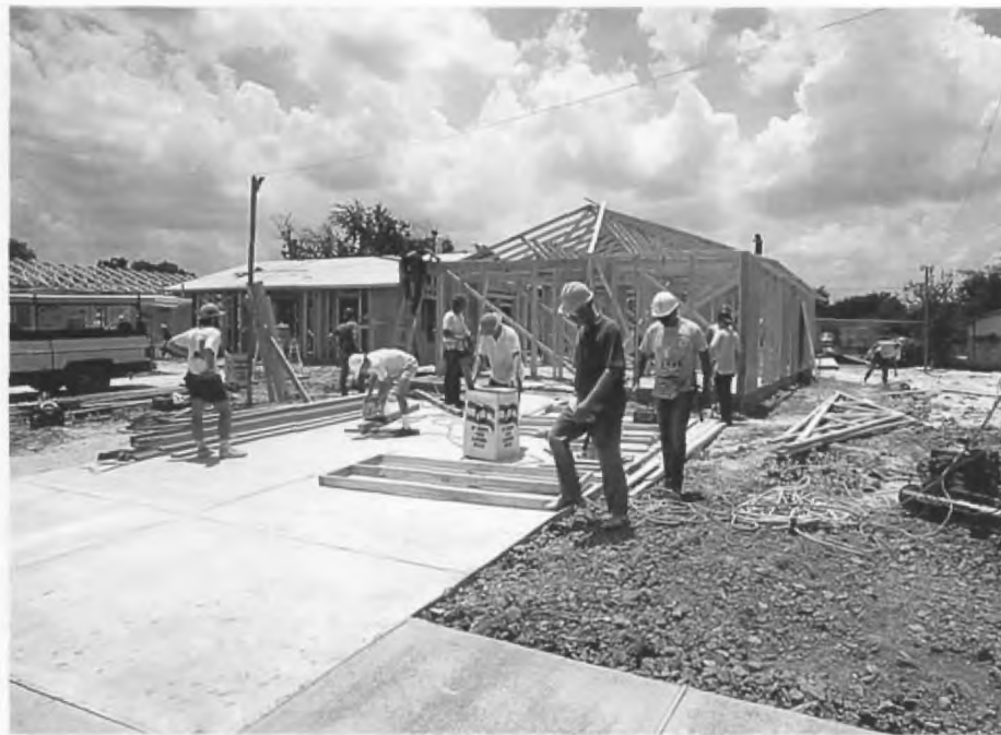
House raising, Habitat for Humanity, Houston chapter.
