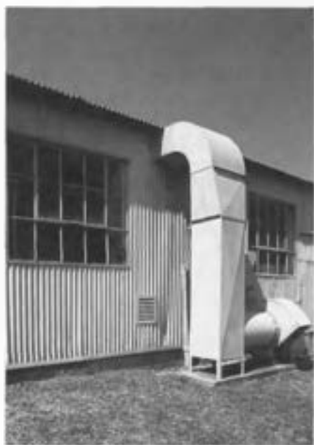
Air-handling unit, General Warehouse and Maintenance Building (now Arts Annex), University of Houston, c. 1946.
