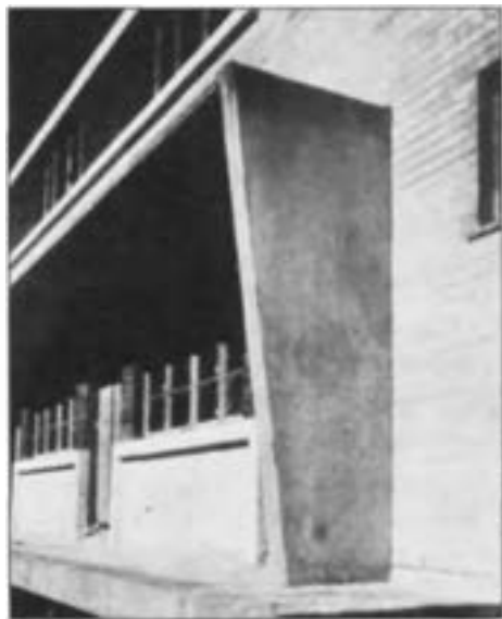
Detail of cast-in-place concrete canopy shielding first-floor window, Allen Parkway Village, 1942. The designing architects, MacKie & Kamrath, ingeniously combined ordinary building materials to give the apartment blocks much richer surface finishes than were customary for U.S.H.A.-built public housing complexes.
