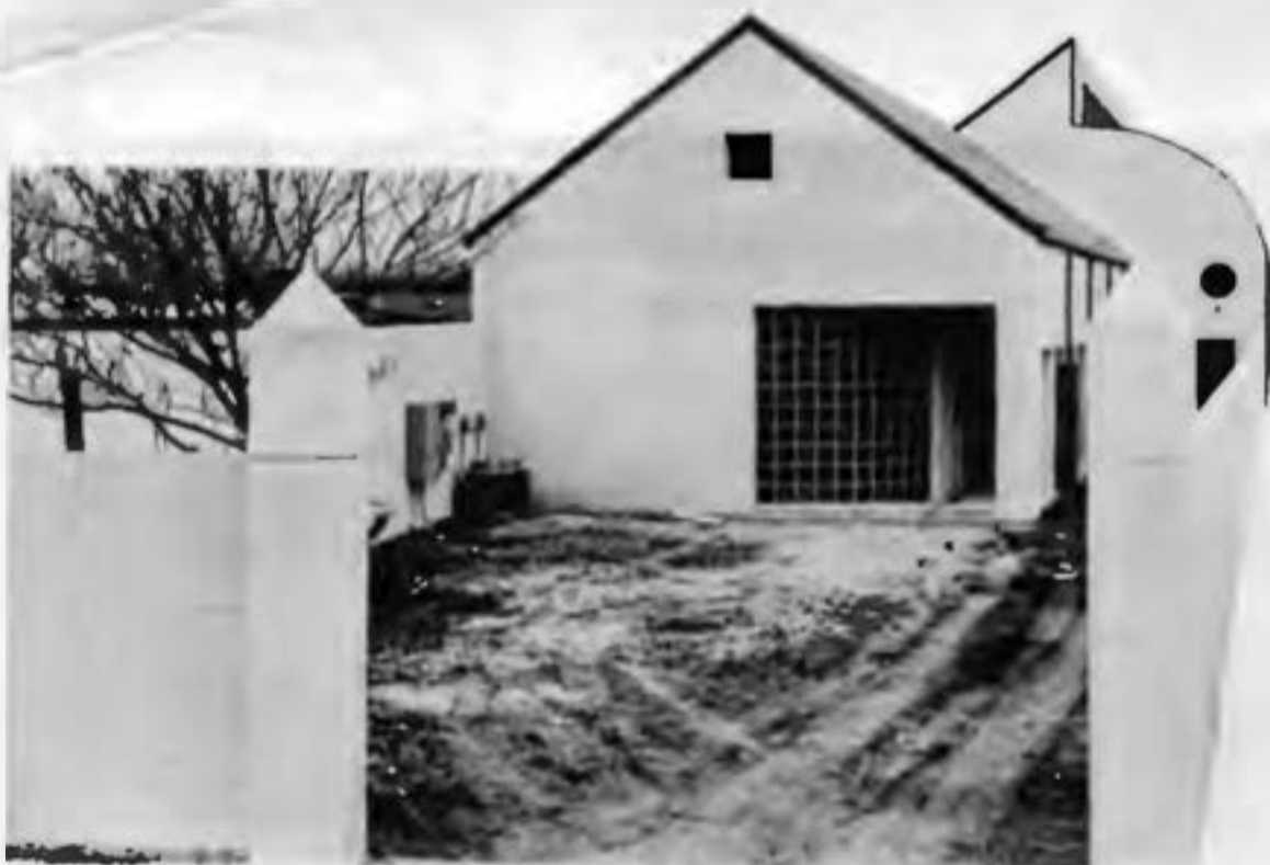
Left: Houston Fine Art Press Building, Carlos Jiménez, 1986 (Photo by Paul Hester). Below: Elevation and sections (courtesy Carlos Jiménez). Bottom: Plan (courtesy Carlos Jiménez)
