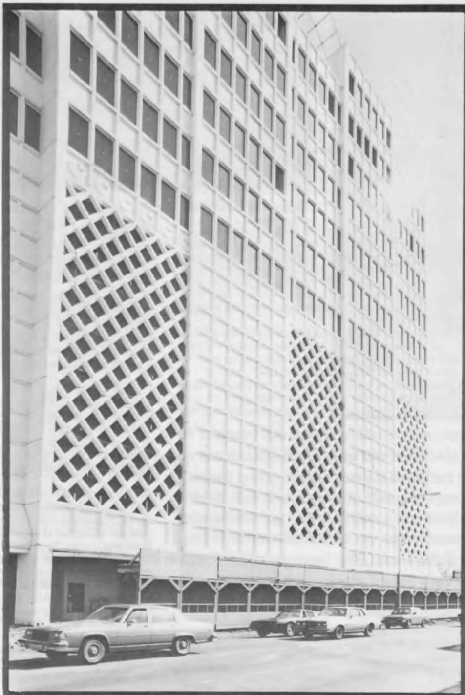
Shepherd Place, under construction, Lloyd E. Pape and Ambrose and McEnany, architects. A project begun before the development ordinance went into effect. (Photo by Paul Hester)
