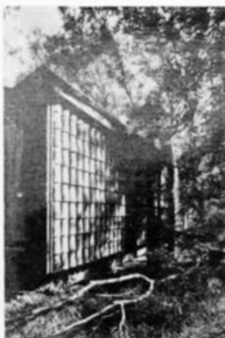
Lyne House, detail of tile-hung exterior wall (Photo by Paul Hester).
