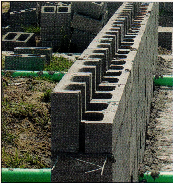
FIGURE 3. Lacking locally available L-blocks, a builder in Louisiana resorted to cutting standard-size blocks to create the slab form. While effective, this work-around increased the cost of completion.
