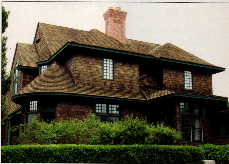
FIGURE 1. A Nantucket dormer provides the headroom of a shed dormer with visual appeal of two doghouse dormers. Here, it is used to define one side of an entire house, where a plain shed dormer would have been too boxy.
