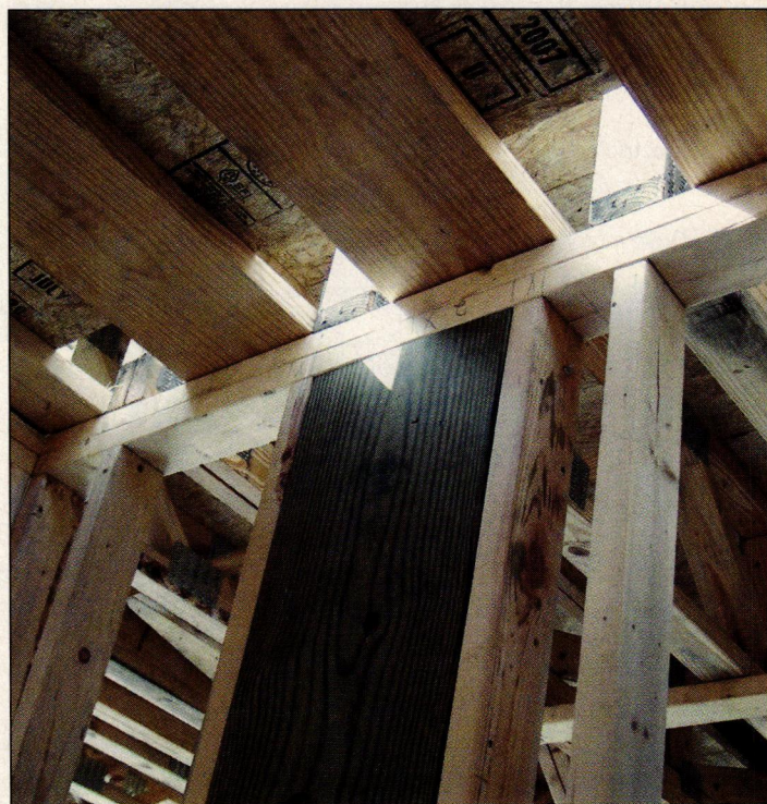
The elevator's steel rail rides on a "rail header" framed out of 2x12s laminated together with glue and screws, and banded by a pair of 2x4s. Note: Temporary planks and decking are required fall protection during construction.
