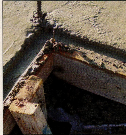
FIGURE 3. During the 2004 hurricanes, wind-driven rain and excessive ground-level runoff leaked under exterior doors and through the cold joint at the base of CMU walls. Mercedes Homes solved these issues during slab forming: A recess formed in the slab, in conjunction with out-swing doors, limits water intrusion beneath doors (above). At the perimeter of the slab, a recessed step provides a key for the poured walls that effectively cuts off a direct pathway for ground-level water (right).
