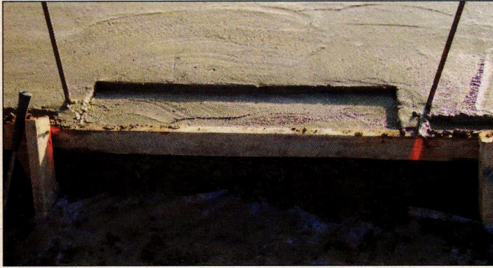
FIGURE 3. During the 2004 hurricanes, wind-driven rain and excessive ground-level runoff leaked under exterior doors and through the cold joint at the base of CMU walls. Mercedes Homes solved these issues during slab forming: A recess formed in the slab, in conjunction with out-swing doors, limits water intrusion beneath doors (above). At the perimeter of the slab, a recessed step provides a key for the poured walls that effectively cuts off a direct pathway for ground-level water (right).
