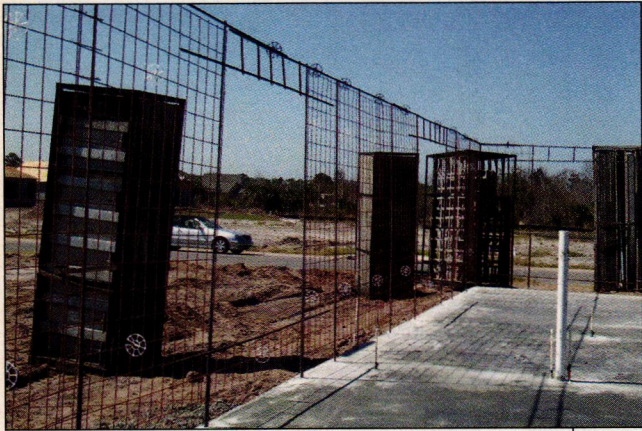
FIGURE 2. The heart of the Solid Wall System (SWS) is a steel reinforcing cage of 6x6x1/8-inch "road mesh" combined with vertical 5/8-inch reinforcing bars placed at 4-foot intervals (above). The cage is specifically designed to evenly distribute lateral wind loads and minimize point stresses imposed by missile impacts, which can lead to failure. The steel cage also connects to steel in the footings. Wet-set tie-downs (hurricane straps) are embedded every 2 feet in the concrete as the walls are poured, providing a continuous path to resist uplift.
