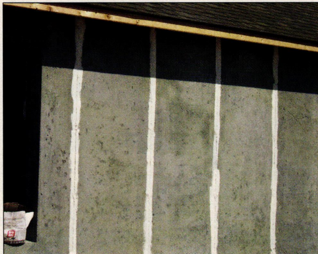
FIGURE 4. Form joints and snap ties are possible water entry points for wind-driven moisture. Applying sealant to these potential pathways is a simple, effective way to prevent water damage to the interior.
