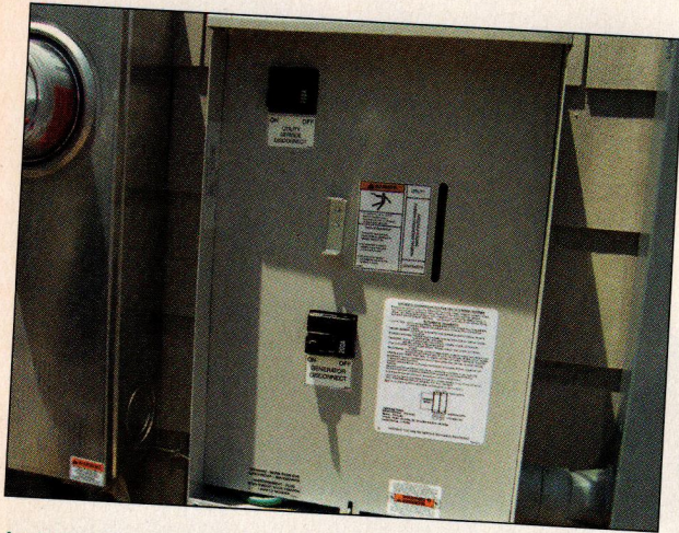
An integrated double-pole, double-throw transfer switch safely disconnects house circuits from the utility before connecting them to the generator, while maintaining a continuous ground for both power sources. The switch may be manual (above) or automatic (right).
