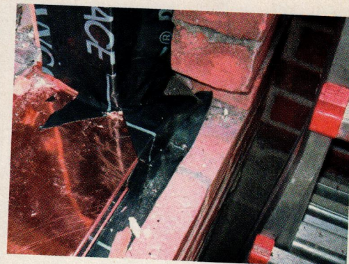
FIGURE 3. The author uses a metal brake to form a copper pan (left). All windows eventually leak, but the pan will capture the water and allow it to drain to the exterior. The inside of the pan should have an upturned edge to prevent the water from draining to the interior, and the side flashings should lap over the ends of the pan (above).
