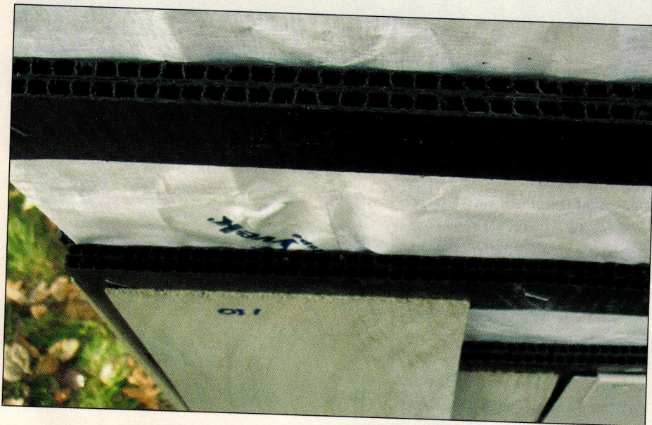
FIGURE 2. Plastic battens have hollow channels that let water and air flow through them. Shown here is the two-ply version of CedarVent, which the author rips to 1 3/8 inches wide to save material and expose more of the shingle back to air.
