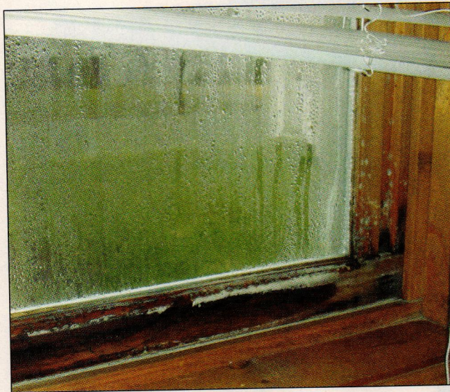
FIGURE 1. High indoor humidity levels, aggravated by a window blind that reduced the drying effect of air circulation, has created a condensation problem that has led to mold growth. In this case, the homeowner's lifestyle lies at the root of the problem, but it's not helped by an ordinary insulated window without warm-edge low-conductive glass.
