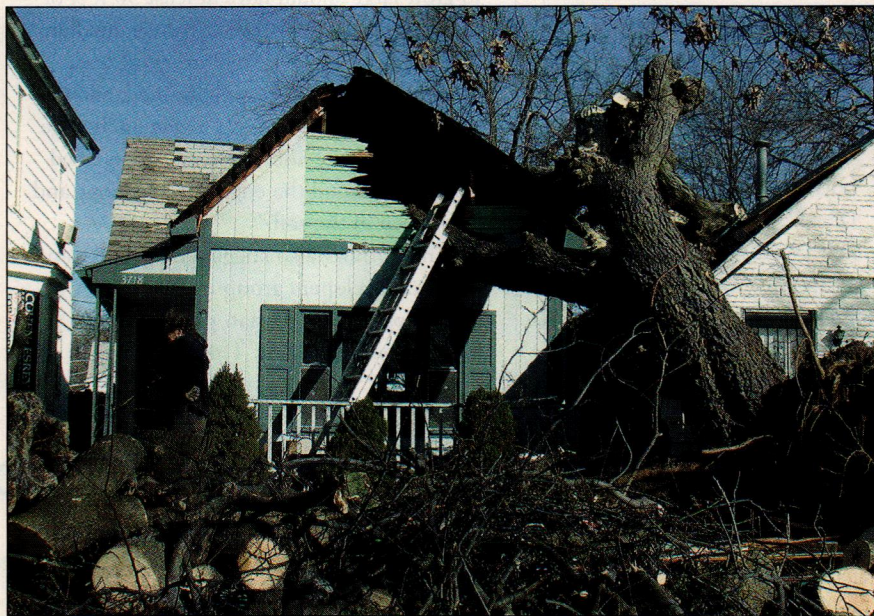
Toppling trees prove to be a leading culprit in damaging houses during high-wind events. Builders and planners seeking to make new communities as hurricane-hardened as their houses have learned to pay attention to the kinds of trees they plant.
