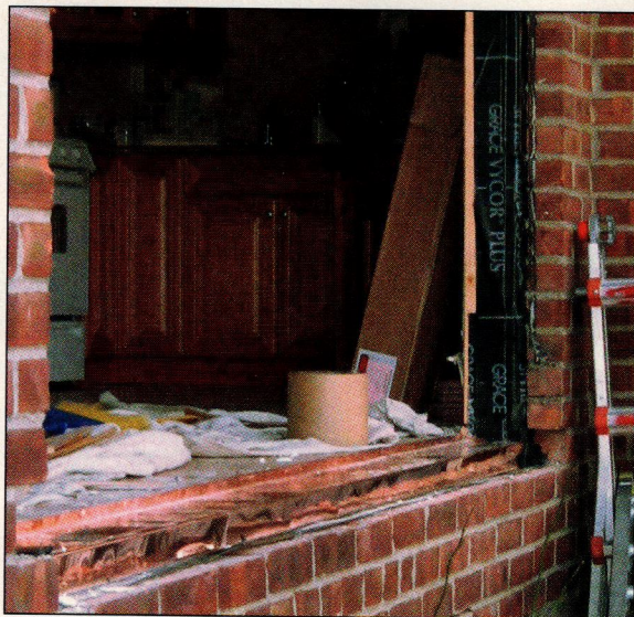
FIGURE 4. The author sandwiches the door's nailing flange in Vycor Plus (above and top right) — one layer hugging the trimmers and a second layer lapping the flange. While sometimes considered a redundancy, this “belt and suspenders” approach provides protection from the hard-driving north-easterly winds that blow across Long Island in winter.
