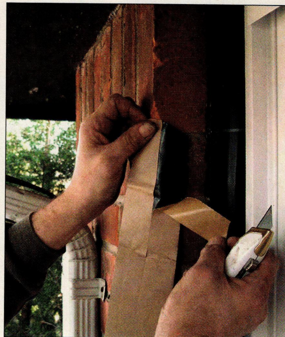
FIGURE 4. The author sandwiches the door's nailing flange in Vycor Plus (above and top right) — one layer hugging the trimmers and a second layer lapping the flange. While sometimes considered a redundancy, this “belt and suspenders” approach provides protection from the hard-driving north-easterly winds that blow across Long Island in winter.
