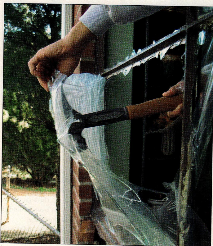
FIGURE 1. Carpet Protection — a strong, self-adhesive plastic film — adheres well to glass (above). When it's applied to both sides of the window, the glass can be broken out without creating a hazard (right).
