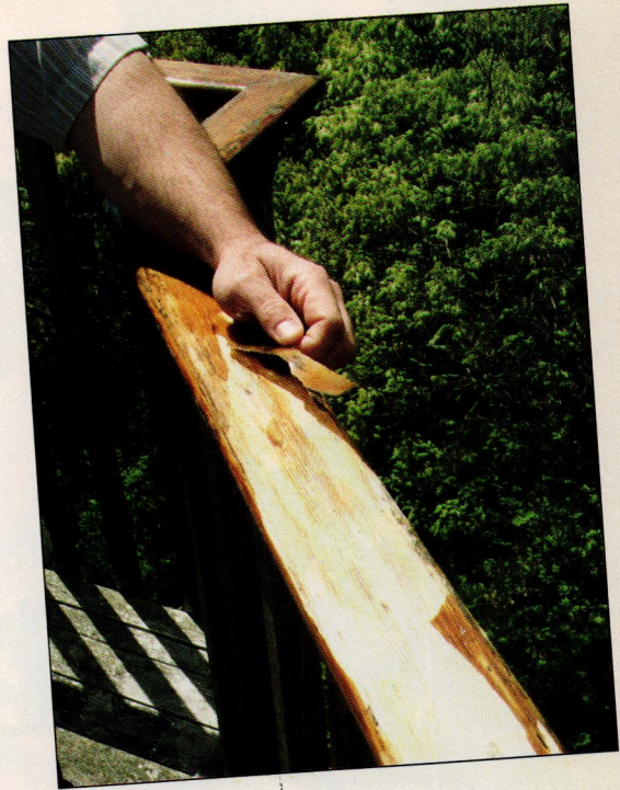
FIGURE 3. The reason boat owners love spar varnish is shown above: a deep, rich, clear coat that repels water and reveals all the beauty of the wood. A finish like this takes 10 to 12 coats, however, and needs continual attention to maintain its good looks. Without a yearly sanding and refreshing, varnish fails by yellowing and peeling (right). When that happens, it's time for sanding back to bare wood and starting over.
