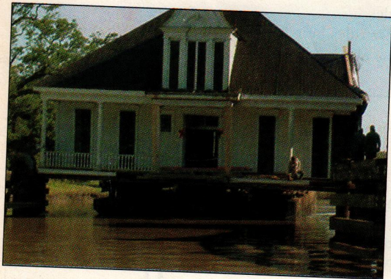
FIGURE 4. On its way to Lake Pontchartrain and eventually to its resting place on Lakeshore Drive in Mandeville, Justine, supported on a grid of steel, is pulled upriver on a barge (above). At the Mandeville seawall (right), the entire home is rolled off the barge and towed across the street to the corner of Gerard Street and Lakeshore Drive.
