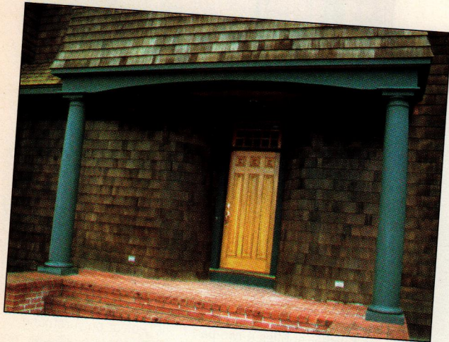
FIGURE 1. Clear finishes last longer when sheltered from direct sun, as in the entry to this Rhode Island home by architect/builder Andrew DiGiammo. The more exposed wood trim has been painted on this house, and wood shingles have received an opaque stain.
