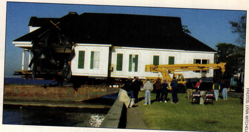
FIGURE 4. On its way to Lake Pontchartrain and eventually to its resting place on Lakeshore Drive in Mandeville, Justine, supported on a grid of steel, is pulled upriver on a barge (above). At the Mandeville seawall (right), the entire home is rolled off the barge and towed across the street to the corner of Gerard Street and Lakeshore Drive.
