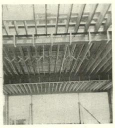
To these horizontal strips were nailed vertical pieces, their length being such that they allowed room for another horizontal strip to be nailed below the steel girder. This was done on both sides of the girder.
