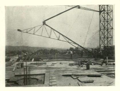
delivers concrete in a practically continuous flow. The job need not be so very large to justify equipment like this sturdy apparatus
