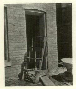
The horizontal braces are set about 1 ft. off the ground so that the upper edge of the brace sets under the first tread. Everything is nailed securely, and the ladder moved about in the open position.
