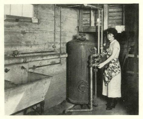
The modern water softener is simple to operate and maintain. Above is a typical Wayne Water Softener at work in the house
