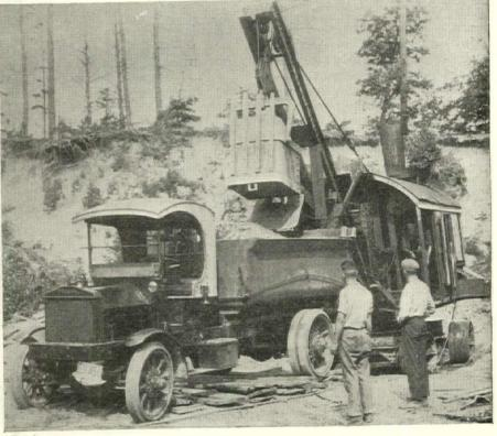
If the jobs are getting too big for the old equipment there are plenty of modern machines to choose from. Here is a typical layout for quick excavating. A few scoops from the giant shovel and the truck is filled. No gang of shovelers to eat up labor estimates through inefficiency
