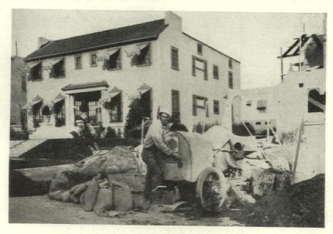
Fig. 2. For speeding the mixer from job to job this one is mounted on rubber tires. The single unit, hooked up to the back of a Ford, may be trailed along at a good speed
