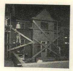
Careless and hastily thrown together stagings are usually unsatisfactory. Here, the structure is insecure and unsteady. In addition, in tearing it down the boards are damaged beyond further use
