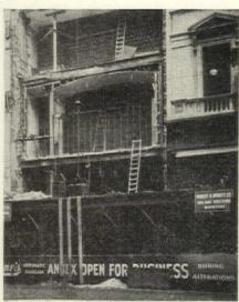
Fig. 5. Here there was no room for a rubbish chute, so a derrick mounted a top the building lowered the debris to the street
