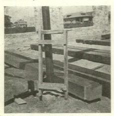
It consists of two 2"x4" legs (D), held together by the 1"x3" braces (B). At the tops of the legs (D) a "V" notch is cut so that two pieces of 1"x4" (A) when tapered at the ends and driven into the notch will be held firmly together. This is the principle of the clamp. The two 1"x4"s (A) need only be tapered at the ends so that they will be held fast when driven into the notches in the tops of the legs.
