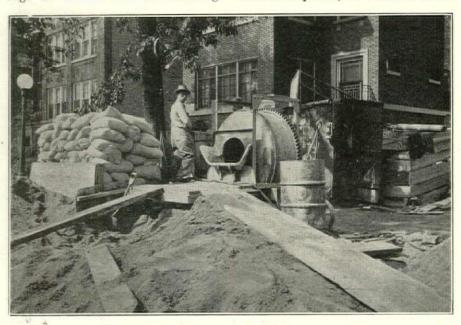
necessary to pour large amounts of concrete continuously. This machine is excellent for small sidewalk jobs and for laying foundations in small buildings but it is hardly possible to use it on a reinforced concrete job where a steady flow and large volume are required. It would take a battery of these to do the work of the machine illustrated in Fig. 3.
