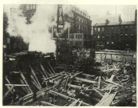
Loading, wheeling and dumping are eliminated in this concrete project. To any point on the job this tower and chuting apparatus
