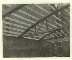
Modern garage buildings are designed to do away with the nuisance of an obstructed floor. Not only garages, but industrial buildings as well, and other types of structures such as dance halls, and sales pavilions require that the floor space be clear, and engineers have provided a simple and comparatively inexpensive type of construction which is especially adapted to the requirements demanded.
