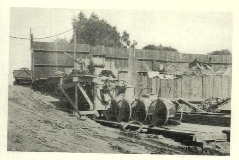
Fig. 3. A two-bag mixer for heavy foundation jobs where a steady flow and large volume of concrete are needed. The installation here is permanent during the erection of the concrete work
