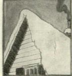
Snow upon the roof of an uninsulated house when occupied melts rapidly due to the heat escaping through the materials from which the roof is built.
