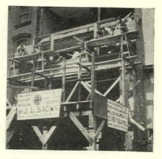
Here, the staging is a maize of timbers put together with little regard for strength or efficiency. Note the unreliable footing for the wooden horses, endangering the workmen's lives unnecessarily
