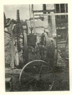
Fig. 3. Hooked to a concrete mixer, this "one-lunger" turns the drum. The mounting structure shown is the chassis of the mixer
