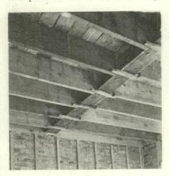
of the I-beam and inasmuch as it was necessary to plaster underneath the beam, some method for holding the lath had to be devised.
