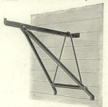
Carpenter Brackets Hook Directly Around Studding and Stand on Two Legs
