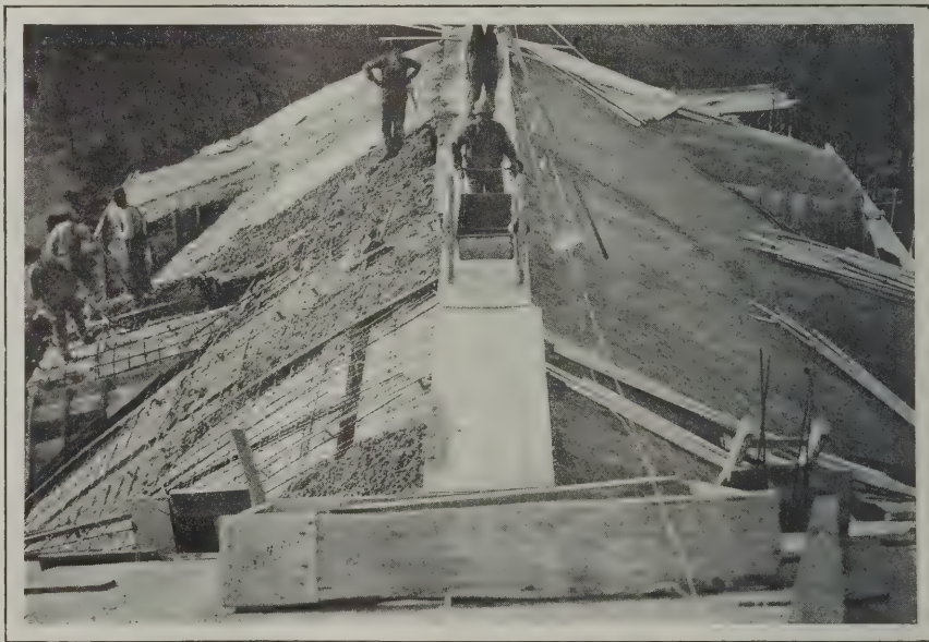
Fig. 3.—Workmen Pouring the Concrete Slab Roof on the North Wing of the Building, One Side Being Already Completed
