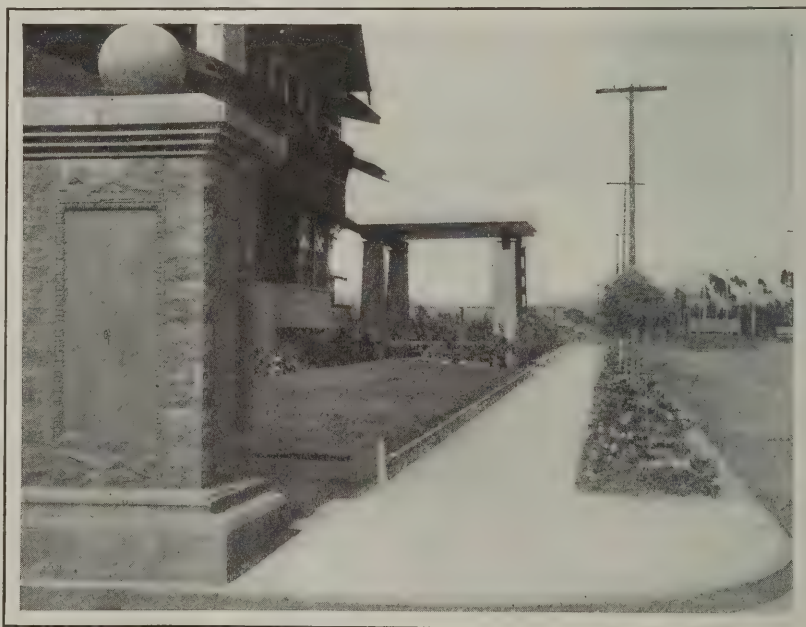
A Concrete Sidewalk at Hollywood, California
