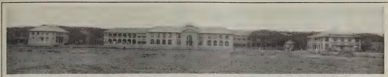
Front View of the Philippine General Hospital of Reinforced Concrete Construction and with Shell Windows
