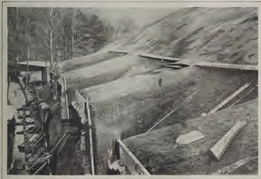
A Unique Roof for a Rather Unique Building.—Fig. 4.—Roof of the South Wing of the Building, Showing Concrete Slab Completed; Also Lazy Lines of the Roof and the Dormer Windows
