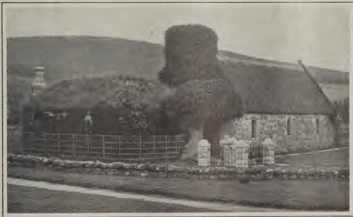
An Interesting Example of Scotch Masonry in which the Walls Are Built of Uncoursed Rubble
