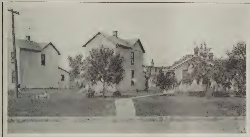
Building Modern Homes for Workingmen—View Showing Generous Yards About the Houses
