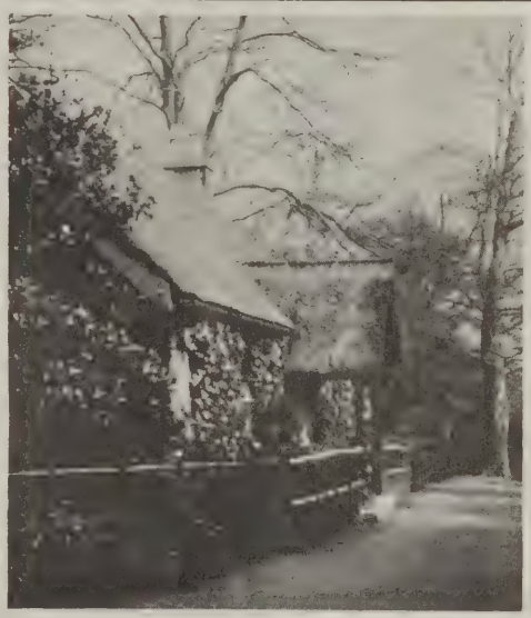
A Porch Having Thatch as Its Roof Covering
