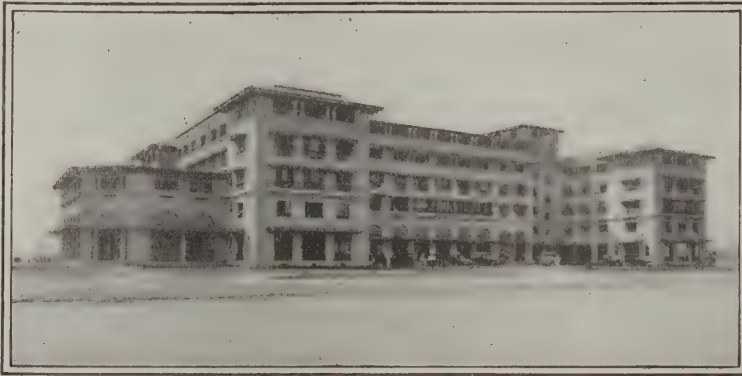
General View of the Completed Building
