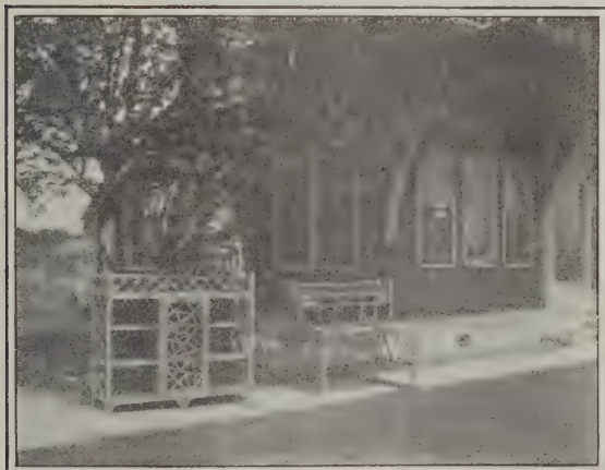
Fig. 1—General View of the Work
