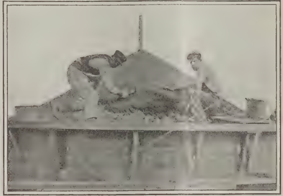
Fig. 3—Covering the Reinforcement with Concrete
