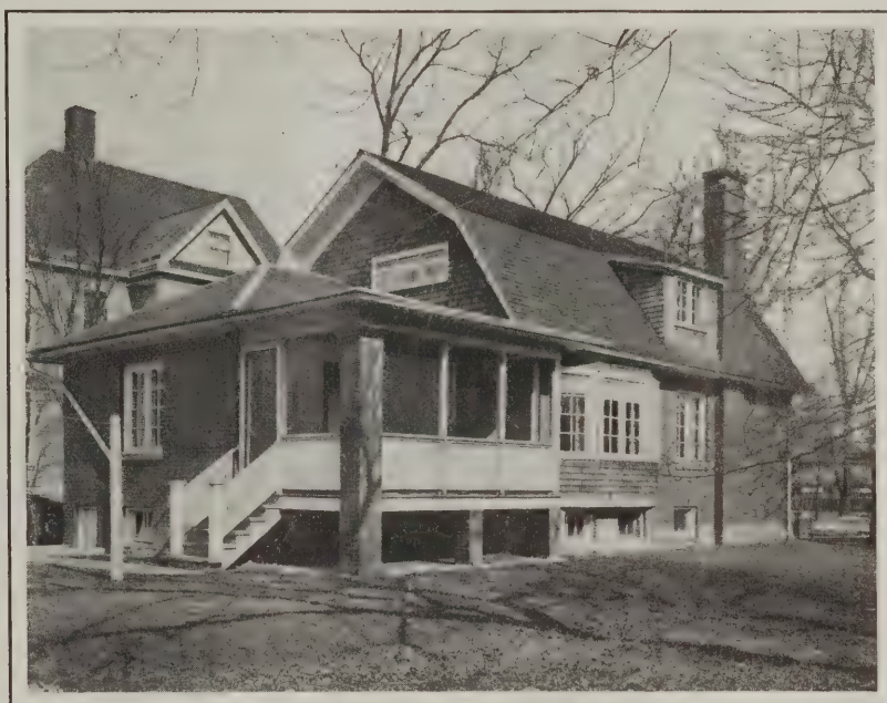
A Rear View of the Cottage Showing Open Side Porch
