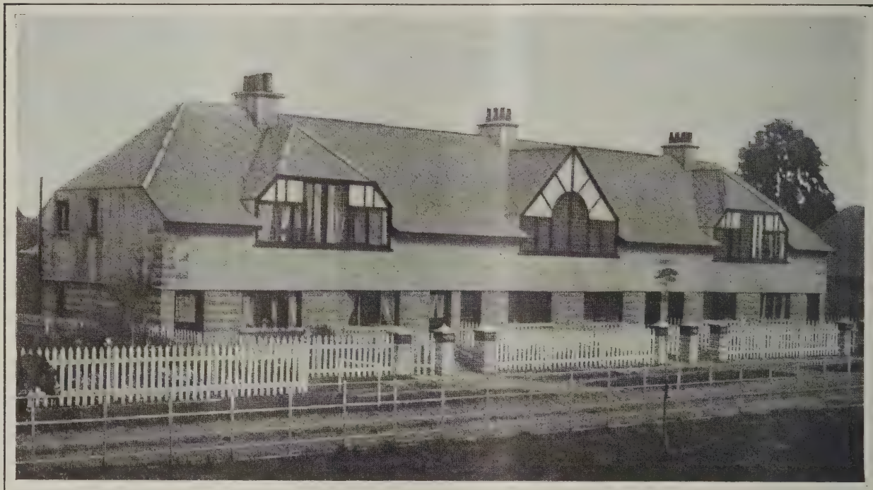
English Cottages of Concrete for Workingmen—View of a Dwelling Having Accommodations for Six Families
