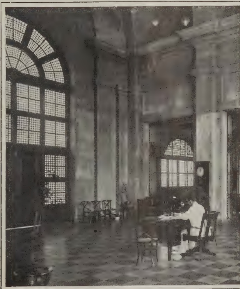
Main Entrance to Philippine General Hospital, Manila, showing Window Sashes Fitted with the Kapas Translucent Shell and Sunlight Effect on Inner Side
