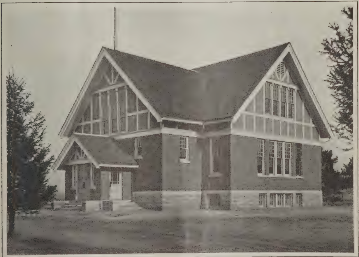
Photographic View of a Modern Two-Room School House at Wayne, Ill.—Architects, Postle & Fischer, 1732 Marquette Building, Chicago, Ill.
