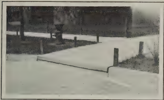
Constructing a Concrete Sidewalk—Showing Provision for Sidewalk Expansion of Curb
