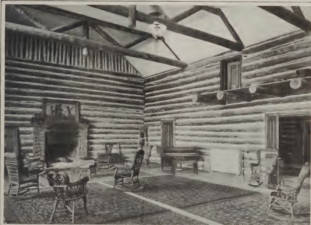
Interior View in Studio Looking Toward the Open Fireplace and Showing Balcony at the Right at Level of Second Floor A Log Cabin Type of Studio Building
