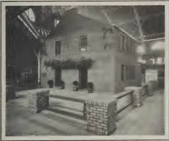
General View of the Prize Brick Cottage at the Clay Products Exposition
