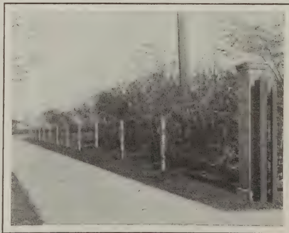
Another Good Example of Sidewalk Construction
