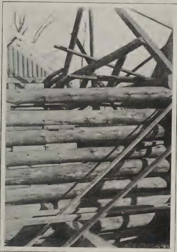
Log Cabin Type of Studio Building—Detail of the Wall Construction, Showing How the Spaces Between the Logs Were Filled with Pieces of Wood Before Calking
