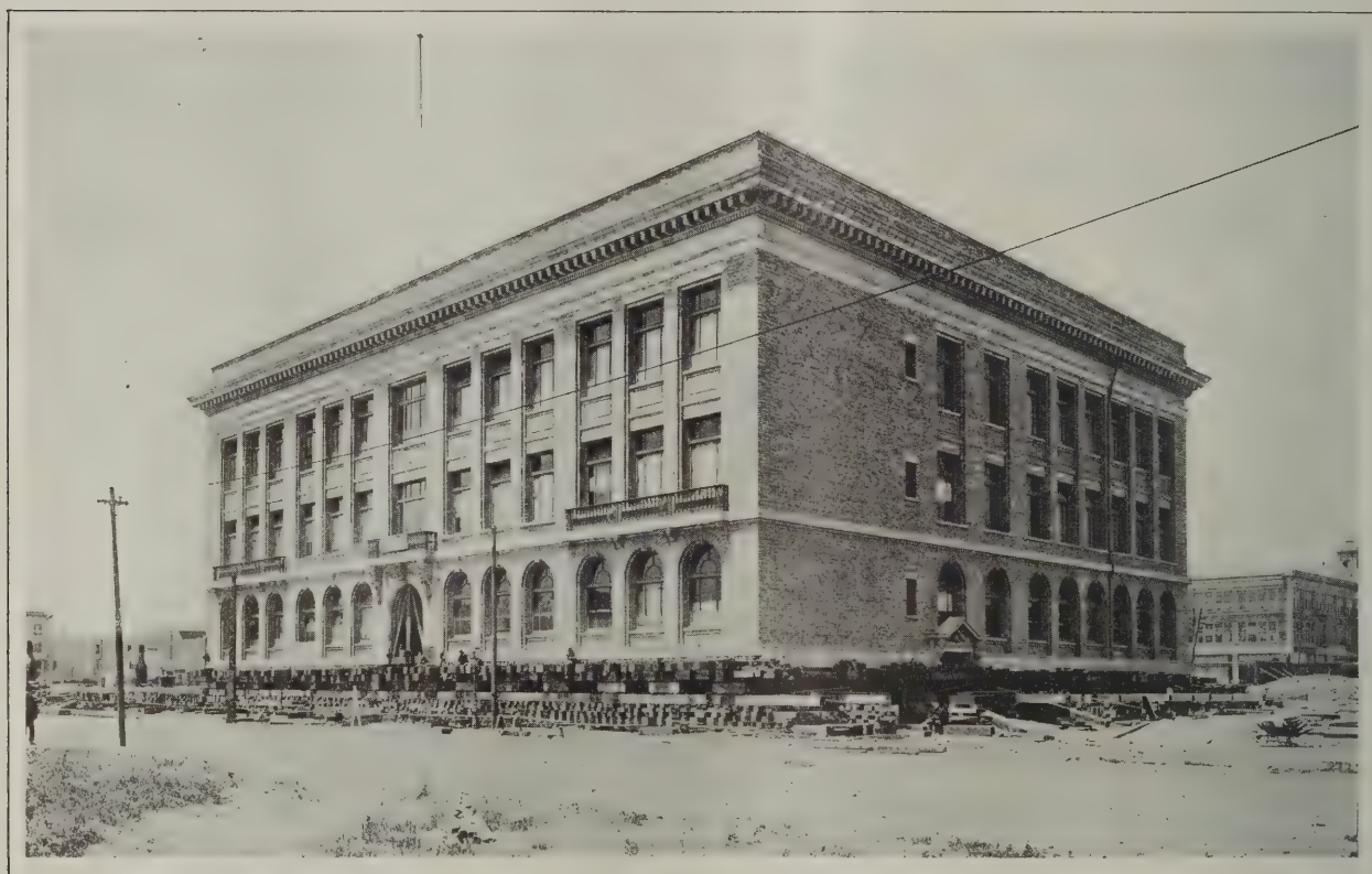
Moving an Eight Thousand-Ton Building—Fig. 1—General View of the Structure Resting on Its Cribbing and Ready for Its Journey
