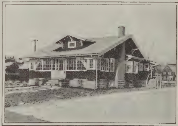
Another view of the house as it appears in winter
