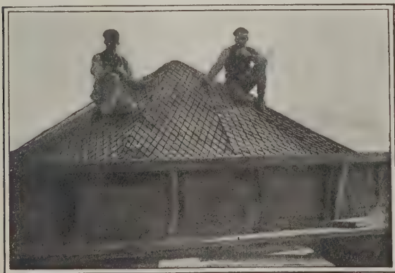
Fig. 2—Roof Reinforcement in Place
