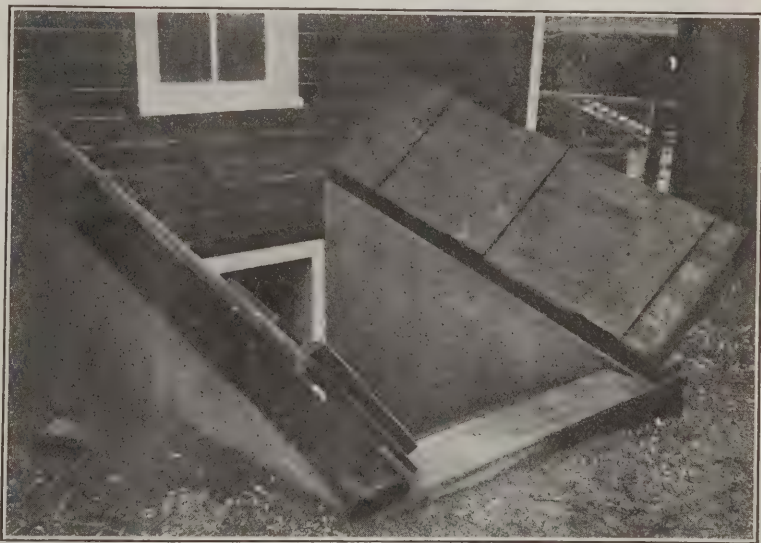
Perspective View Showing Hatchway Completed and the Doors Thrown Back
