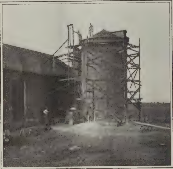
Constructing a Silo Roof of Concrete—Fig. 4—The Silo Completed
