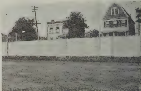
Fig. 11—A Cheap Fence of Concrete Construction
