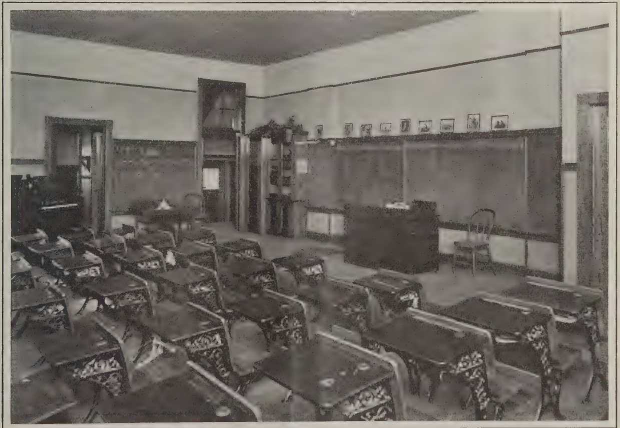
View in Class Room at Right of Partition Looking Toward the Entrance Hall and Showing Arrangement of Desks, Etc.
