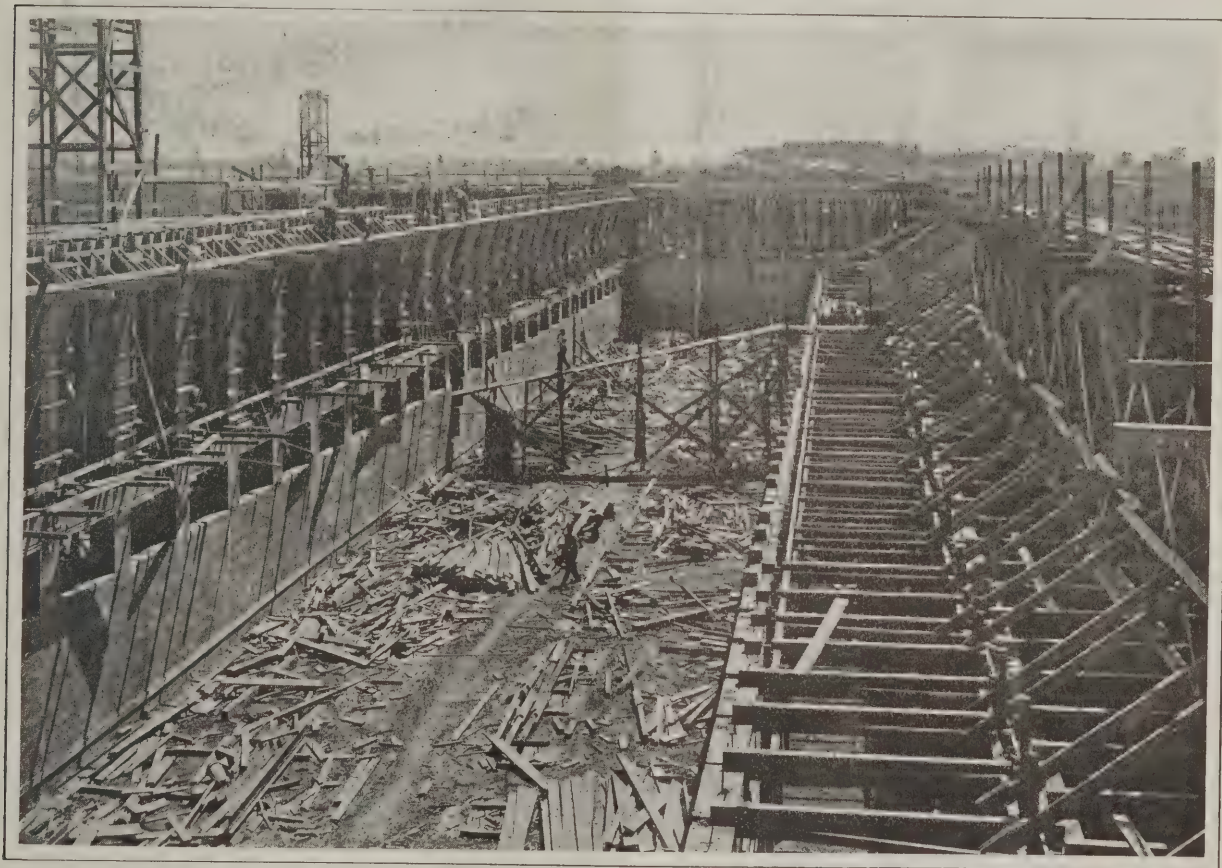
Growth of the Beaver Board Companies—Fig. 1—General View of the Foundations for the New Plant at Thorold, Canada
