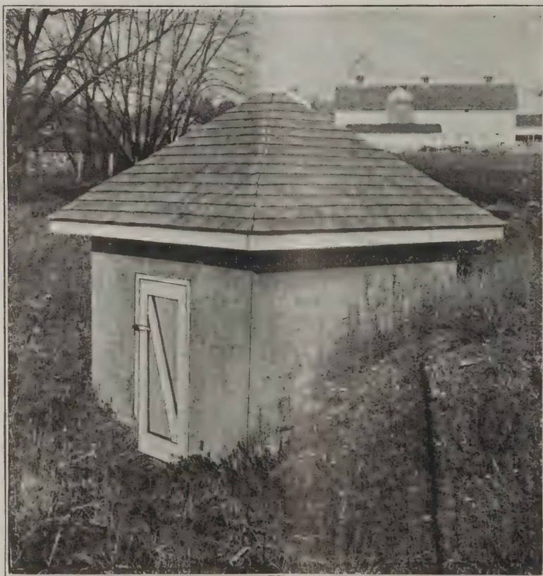
Hydraulic Ram Houses Built of Concrete—A Good Example of Construction on an Illinois Farm
