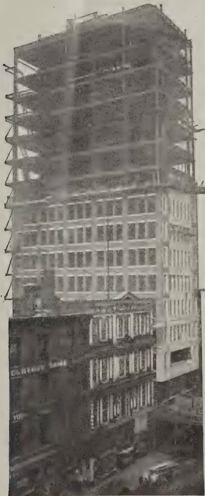
Chicago's New Advertising Building as It Appeared in Process of Construction
