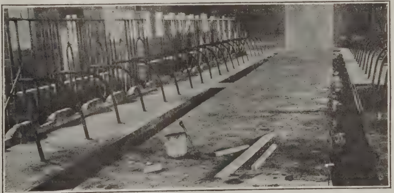
Fig. 2—View of Driveway with Swinging Stanchions, Concrete Mangers and the Two Lines of Drop Gutters
