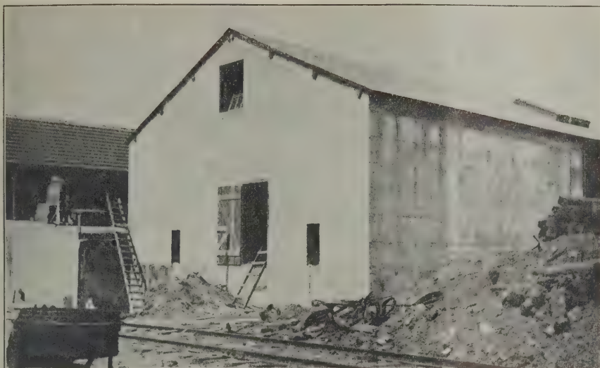
Concrete Barn Built With Blaw Steel Forms
