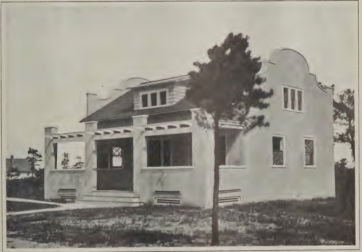
* A Frame Cottage with Exterior of Stucco—Photographic View Showing the Completed Structure
