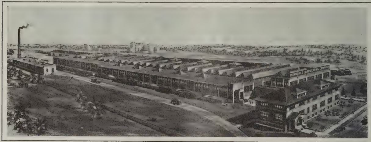
Fig. 1—Bird's-eye View of New Plant of Milwaukee Corrugating Co., at Milwaukee, Wis.
