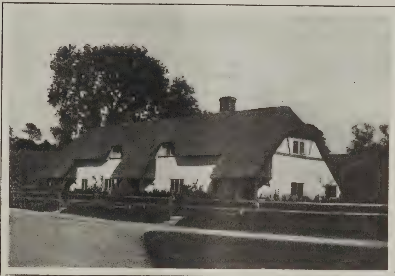
A Dwelling Covered with Thatch Roof Having a Straw Ridge
