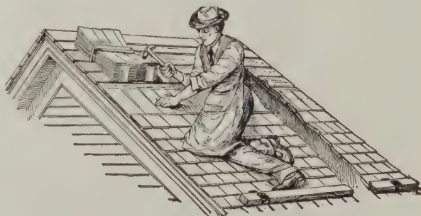
Fig. 4—Showing the Application of Scaffold Bracket on a Roof
