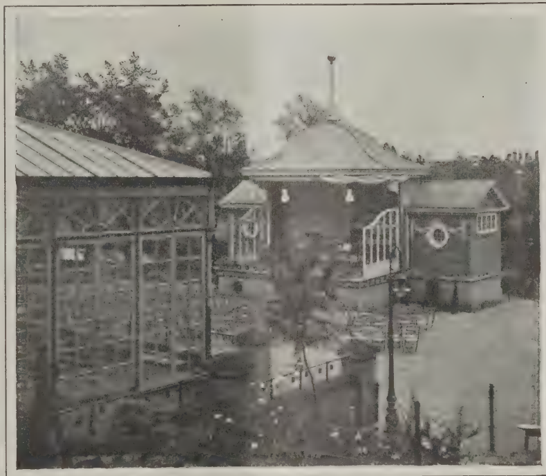
Details of Construction for a Band Stand—Fig. 1—General View of the Completed Structure with Glass Enclosed "Shelter" in the Foreground
