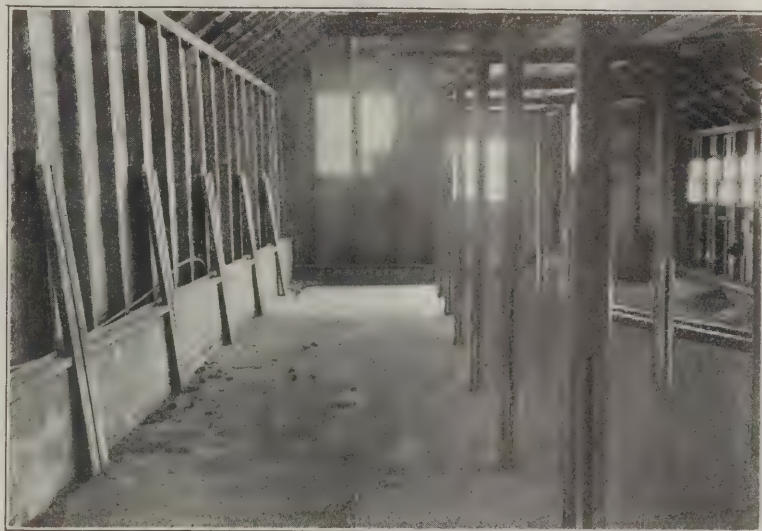
Concrete Hog-House with "Wallow" at the Farther End
