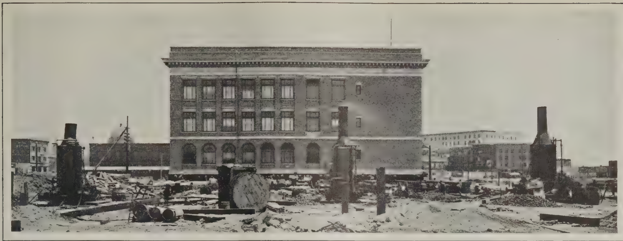
Moving an Eight Thousand-Ton Building—Fig. 2—Looking Toward One End of the School-house with the Donkey Engines Ready for Hauling in the Foreground
