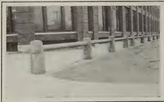
Constructing a Concrete Sidewalk—The Effect of a Well-laid Walk with Attractive Surroundings
