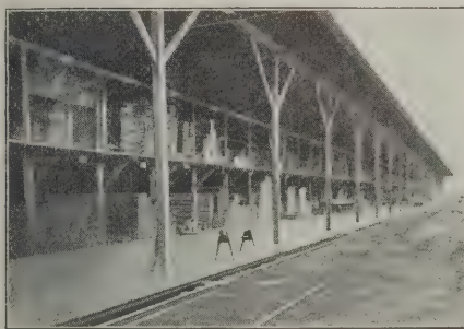
Finishing Lumber, Shed No. 1
