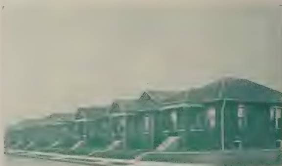
Part of a row of 24 brick cottages erected by Tissier Bros. at East St. Louis, Ill. These Cottages are all covered with Rex-tile Shingles
