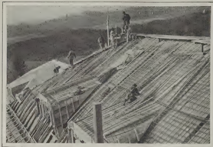
A Unique Roof for a Rather Unique Building—Fig. 2—Portion of the Main Roof Showing Metal Reinforcement in Place and Ready for the Concrete to Be Poured
