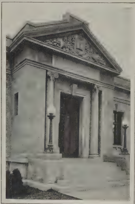
A Detail of the Main Entrance
