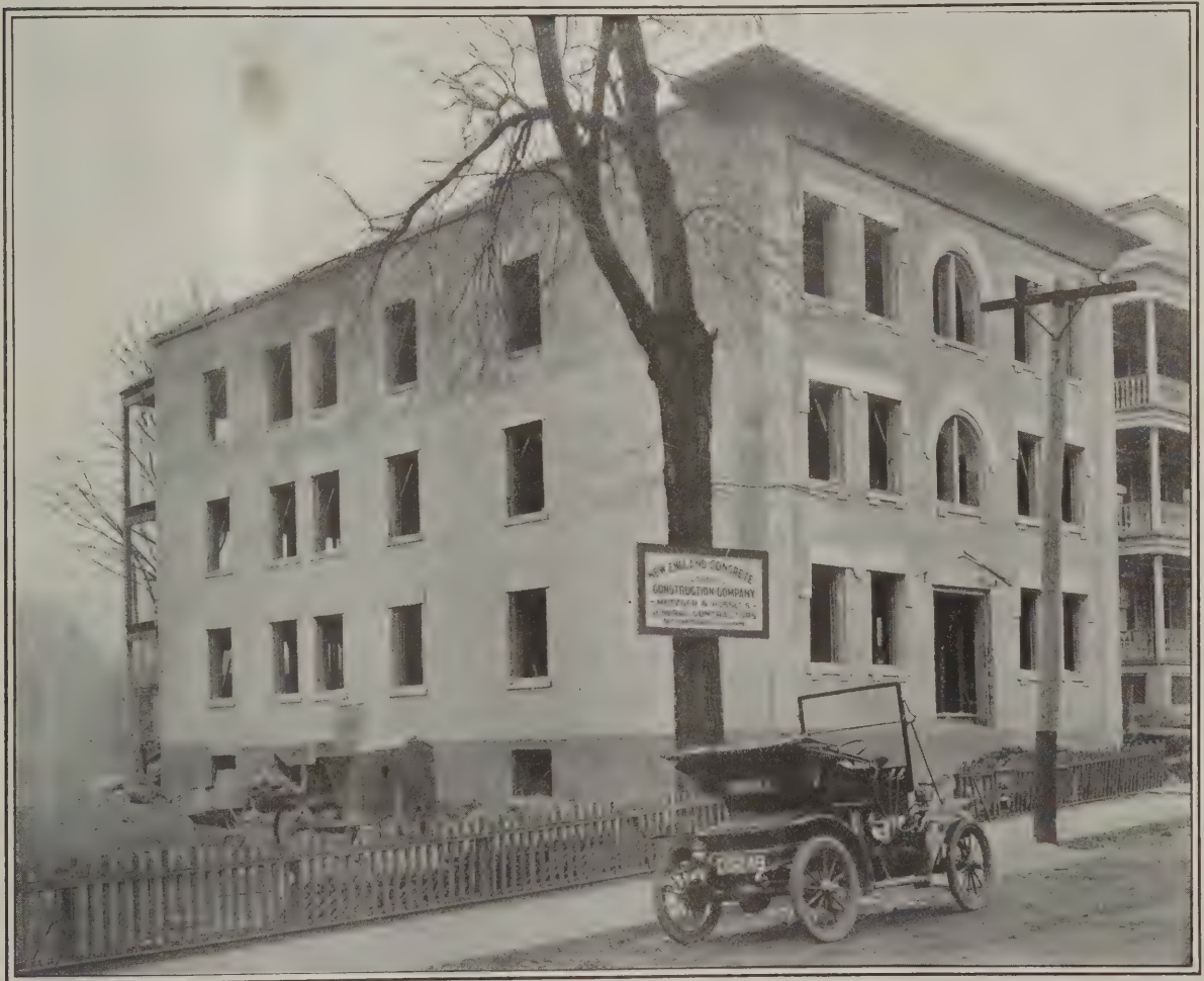
A Six-Family House of Concrete Construction—General View of the Double-Wall Concrete Apartment House After It Had Been Enclosed and the Roof Put On
