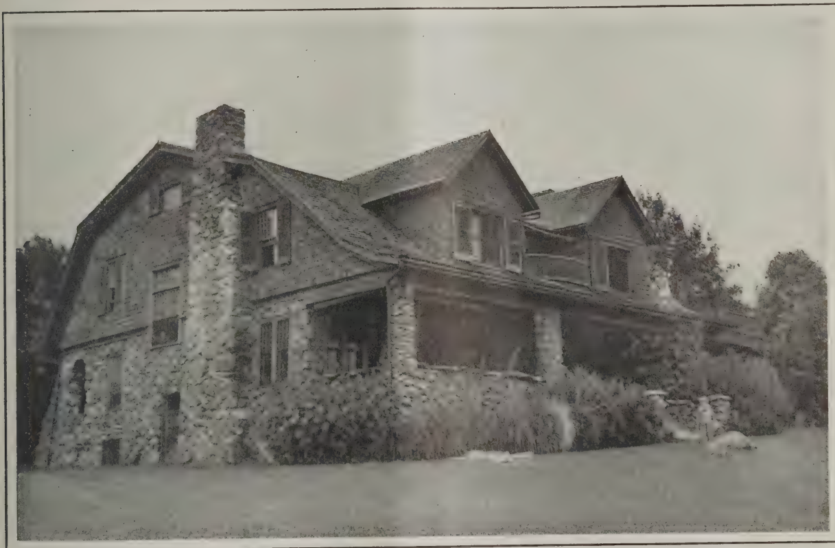
A Stone and Frame House in the Blue Ridge Mountains—Miss H. G. Brouse, Architect, Washington, D. C.
