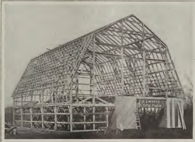
Economy in Farm Building Construction—General View of the Framing
