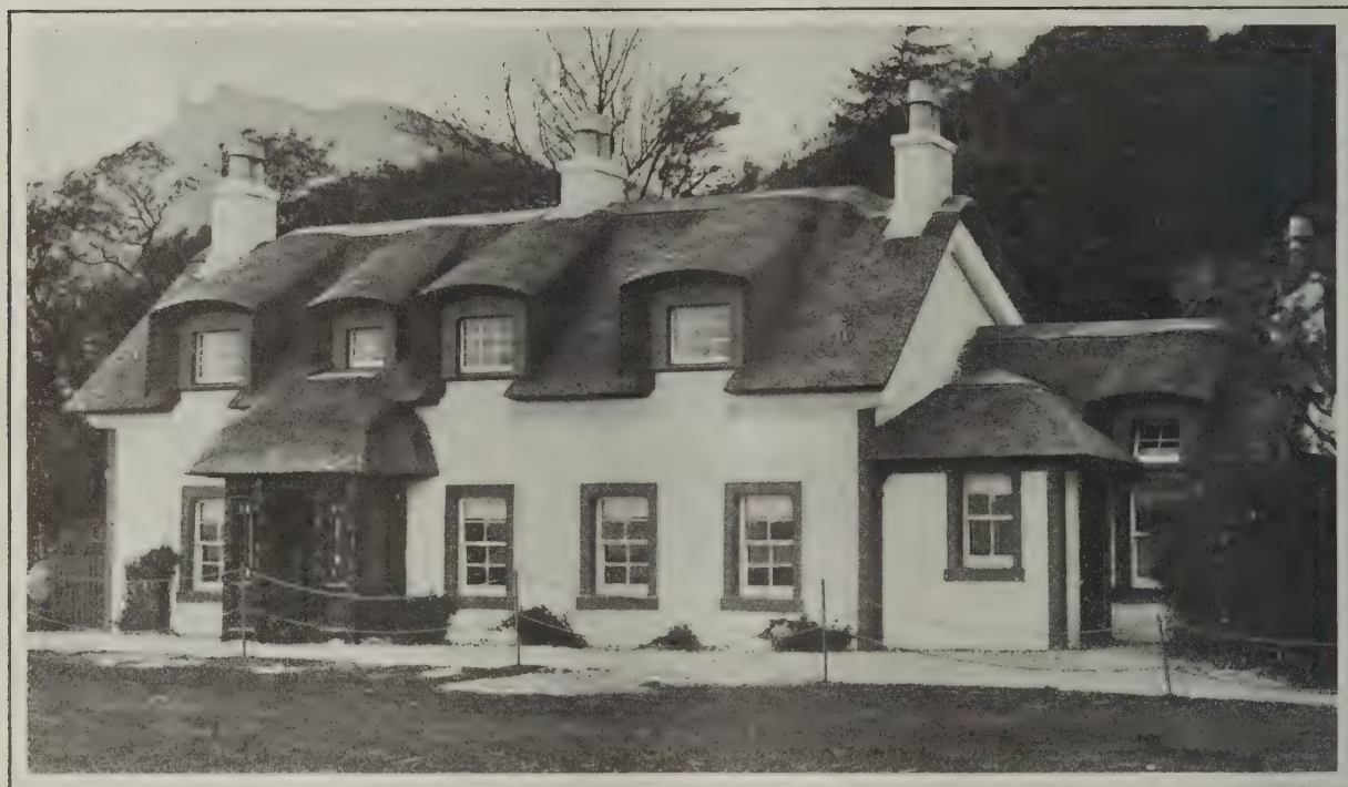
Something About Thatch Roofs for Houses—An Example of a Thatched Dormer Roof Where the Verge Is Carried on an Oversailing Course Formed on the Gable
