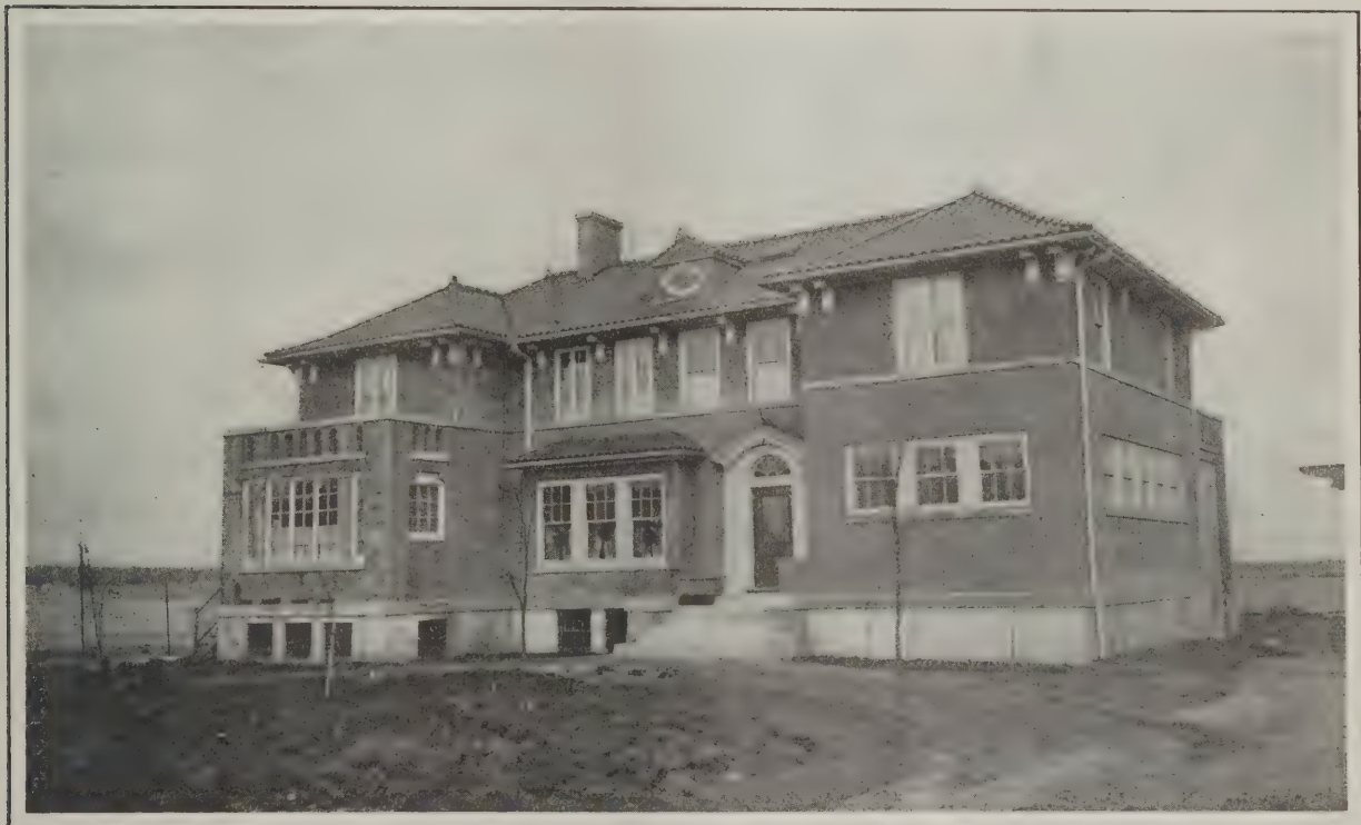
Front View of Dwelling House Having Moving Picture Theatre, with the Waters of Long Island Sound Seen in the background
