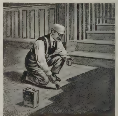
Fig. 16—Giving a floor a varnish finish
