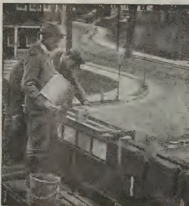
Making ready to insert the floor beams.
