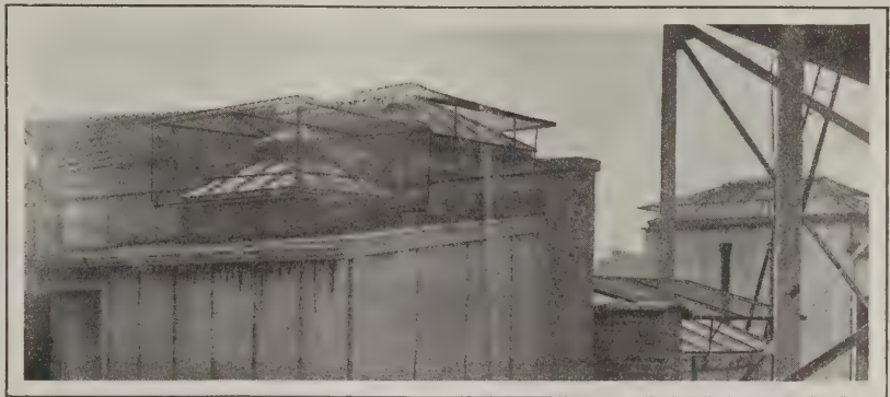
View Showing Skylights Protected by Wire Guards
