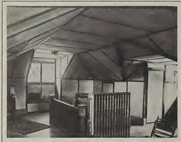
Some Applications of Plastergon Wall Board—Fig. 4—Showing Treatment of an Attic
