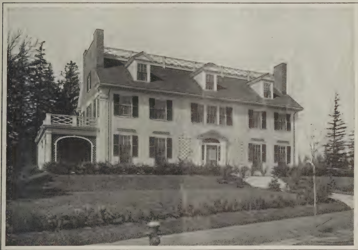
Heating a Country House by Combination System—Photographic View of Residence of Dr. Charles F. Painter at Newton, Mass.
