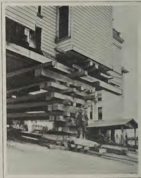
A Close View of One of the Piles of Cribbing A Most Unusual House Moving Operation
