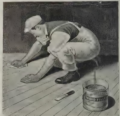
Modern Floor Finishing. Fig. 15—Filling the pores of the wood
