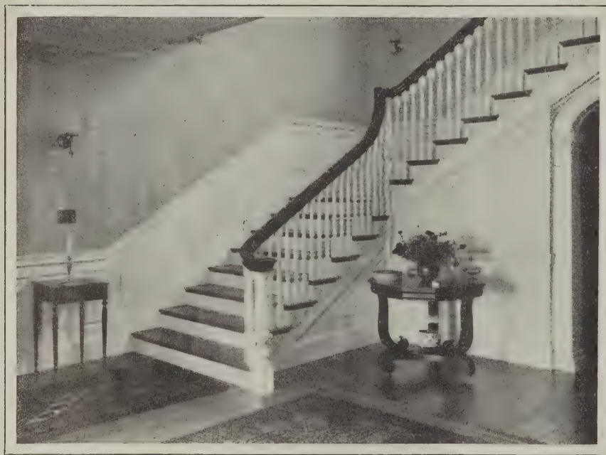
Heating a Country House by a Combination System—View in Main Hall, looking toward the Stairs
