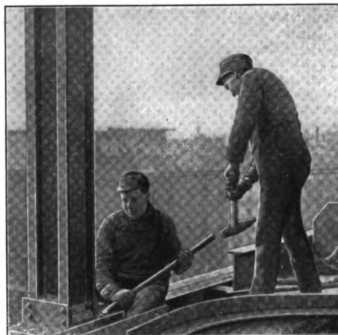
Fig. 2.—Cutting Off Rivet Heads at Foot of Column.
