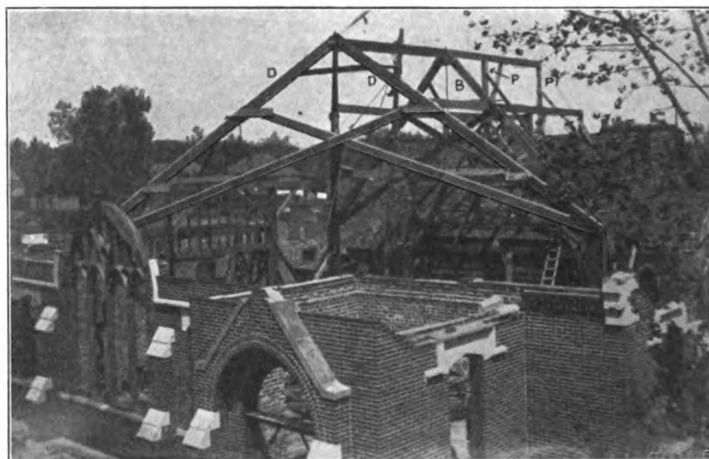
Fig. 12.—Showing Diagonal Truss Over a Church Having Three Arms of Equal Width and Three Gables.
