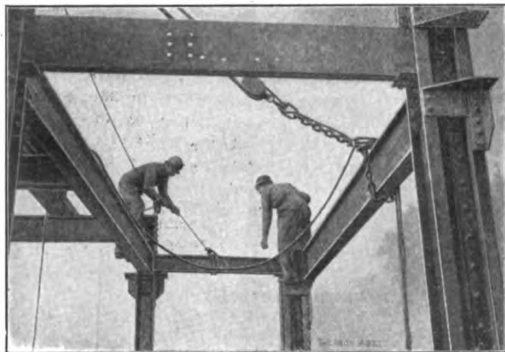
Fig. 3.—Getting Ready to Lower Beam.
