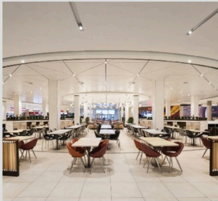
Eventscape: Custom Ceiling Panels eventscape.com For this mall in Canada, Eventscape engineered, fabricated, and installed a 6,000-square-foot ceiling containing 256 triangular panels with integrated lighting. The result is a sparkling display of lights throughout the space.
