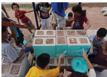
Construction was completed almost entirely by the students of the workshop along with the help of neighbors who spontaneously joined in during the process.
