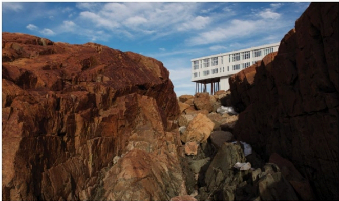
Steel stilts hold up an end of the building that juts out over a rocky promontory. The form references fishing stages that are common in the area.
