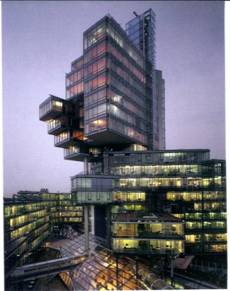
Norddeutsche Landesbank, designed by Behnisch Architekten and Transsolar Climate Engineering, in Hannover, Germany. Photo by Roland Halbe.
