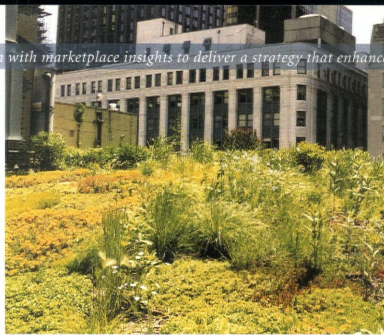
City Hall's green roof (above) has blossomed since 2000.
