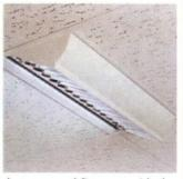
fluorescent lamps in a 2-ft.-long recessed fixture provide the punch of a 500W tungsten halogen. The adjustable, semi-recessed design conceals the reflector aperture from normal view and evenly illuminates the entire wall.
