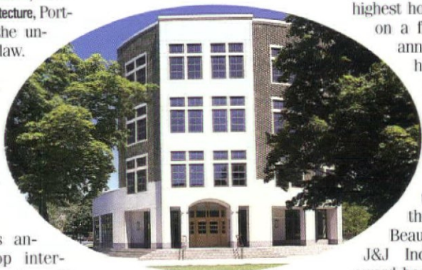
The Princeton University Computer Science Building (above), designed by R.M. Klimont & Frances Halsband Architects, received a 1994 Honor Award from the AIA.
