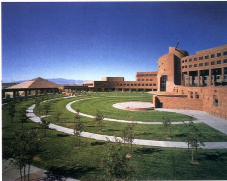
The Clark County Government Center is a desert oasis on the outskirts of Las Vegas. C.W. Fentress J.H. Bradburn and Associates embraced the County's directive that "the building can be more than bricks and mortar," massing the building around a great circle to create a County Courtyard and amphitheater (above). The Center derives its inspiration from the desert environment for its sandstone construction, a pyramid that houses the employee cafeteria, and a kiva that doubles as the central rotunda for the structure (opposite).
