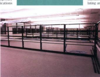
One technique to avoid furniture-related cabling problems is to specify "wiring friendly" center-spine walls that can be put in place, without fabric panels, immediately after carpeting is placed. This installation (above) shows a third-party-manufactured spine wall that has been wired with both electrical and telecommunications wire prior to the commencement of furniture assembly. Custom bracketry establishes compatibility with the fur-
