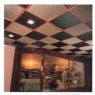
Hunter Douglas's GA-2000 Super Perforated Metal Ceiling features threedimensional geometric shapes, various perforation patterns and vibrant colors that allow a multitude of ceiling possibilities. GA-2000 Super Perforated Ceilings also possess excellent acoustical properties.
