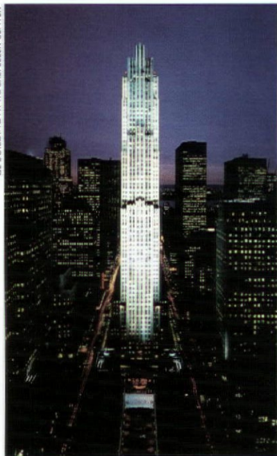
GE BUILDING AT ROCKEFELLER CENTER
