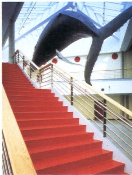
A one-piece rubber flooring stair tread and riser system makes level changes exciting yet safe beside a breaching humpback whale at the Baltimore Aquarium (above), designed by Cambridge Seven Architects. Photo courtesy of Preudenberg Building Systems.
