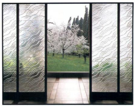
A raised design was incorporated into the Murano glass tiles which create the room's dividing panels. Murano and Formelle glass designs can be used as skylights and privacy panels, and are among Pamio's recent products being distributed through IPI.
